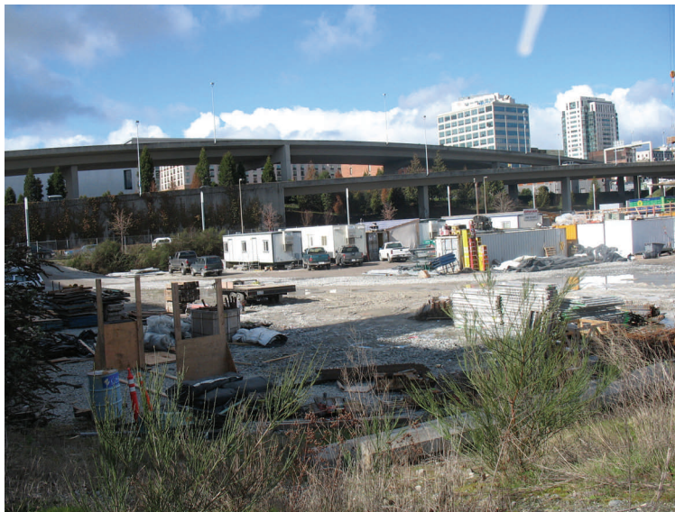
Parcel 3, Site 4 - Facing downtown Tacoma.
