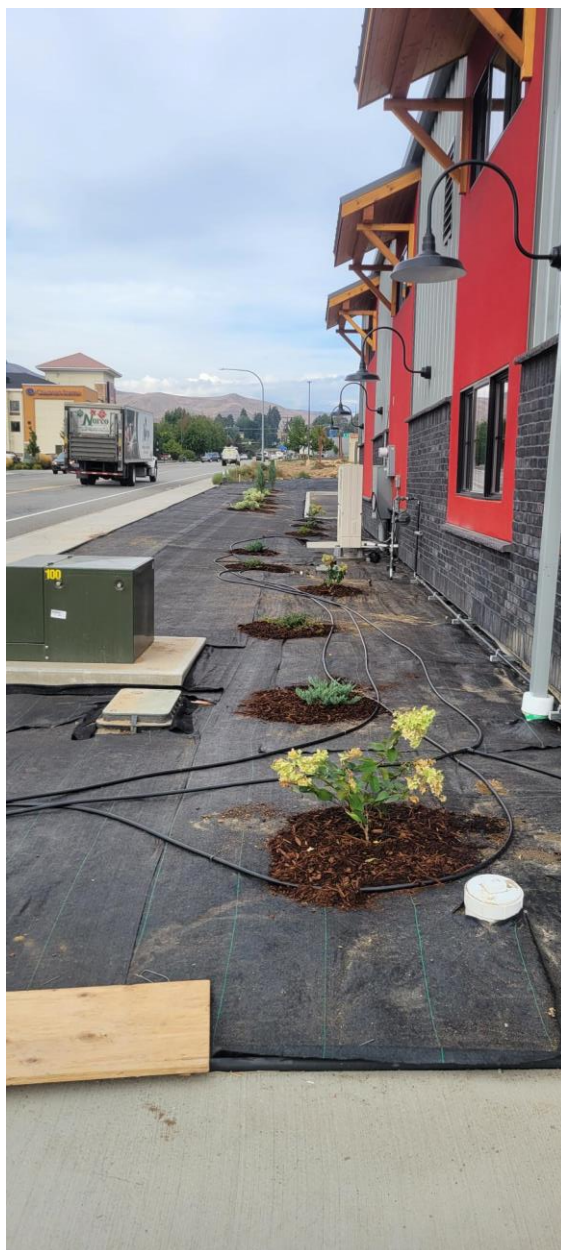
Photograph 8. After installation of the marker material and 6+ inches of clean soils, landscaping areas were further covered with a surface layer of landscaping fabric prior to application of a bark mulch.
