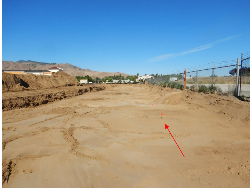
Photograph 3. A 30 ft wide by 200 ft long trench was excavated 30 inches below grade along the northern property line and was compliance tested at 20 sample locations to determine if a clean soil horizon had been reached. Four sample locations did not pass for arsenic only and were marked with orange pin flags (red arrow). However, the average of compliance testing was below MTCA Method A clean up levels.
