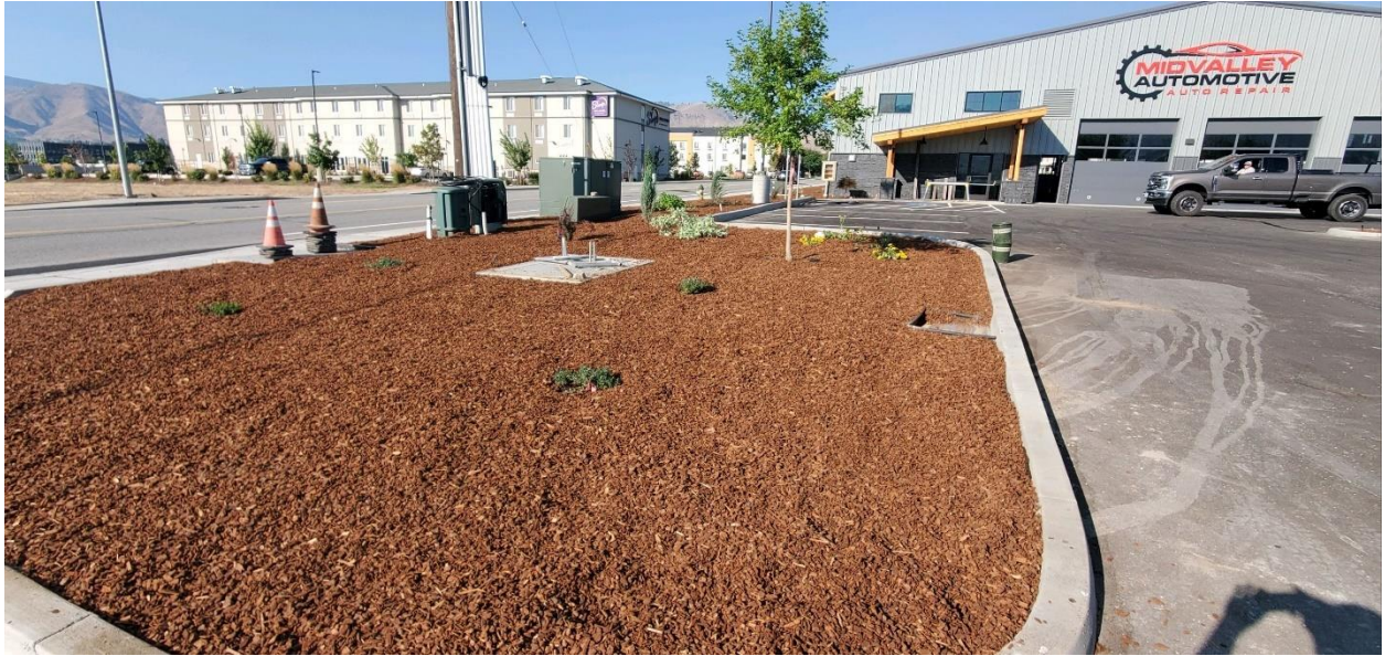
Photograph 10. Final site with soft capped landscaping and hard capped pavement and building.
