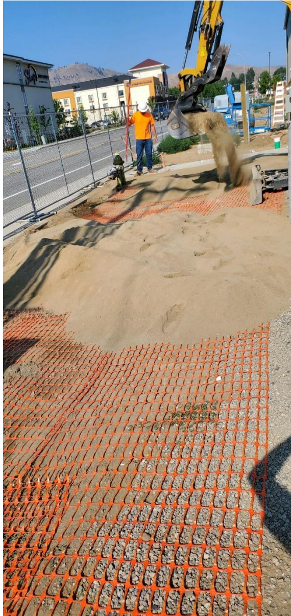
Photograph 6. The marker barrier was capped with 6+ inches of clean soils from the deep excavation clean soil stockpile.
