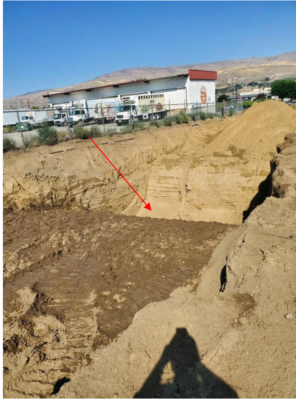
Photograph 4. Clean soils were excavated from below the clean soil horizon within the trench and stockpiled separately from contaminated surface soils. The deep clean soils were lab tested to verify lead and arsenic levels were below MATCA Method A cleanup levels before being exported off-site for stockpile and reuse in the soft cap.
