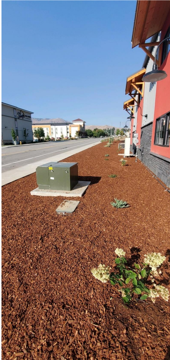
Photograph 9. Several inches of bark mulch were installed over the surface layer of landscaping fabric.
