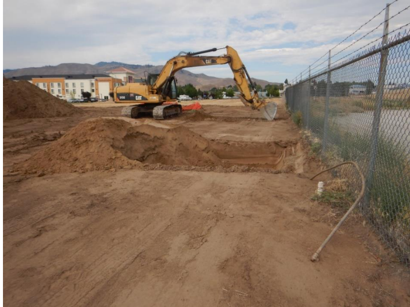
Photograph 1. Seven test pits were excavated along the northern property line.
