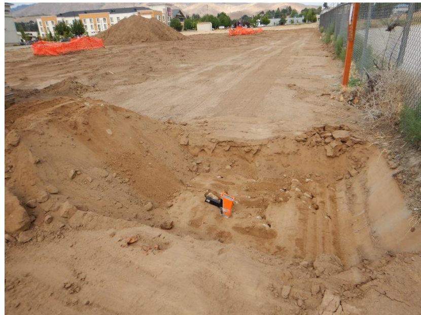
Photograph 2. An XRF was used to evaluate soil contamination at the site.
