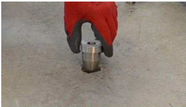
Figure 3. Installing the Drilling Guide.
