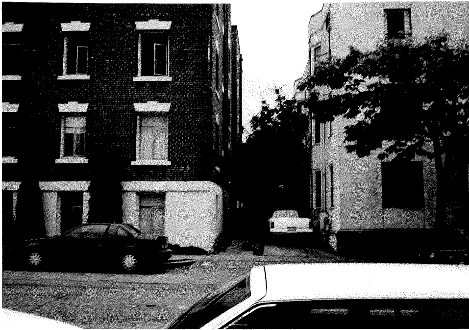
29 View to the north of the Del Roy Apartments on the left of the photograph and the Monterey Apartments on the right.
