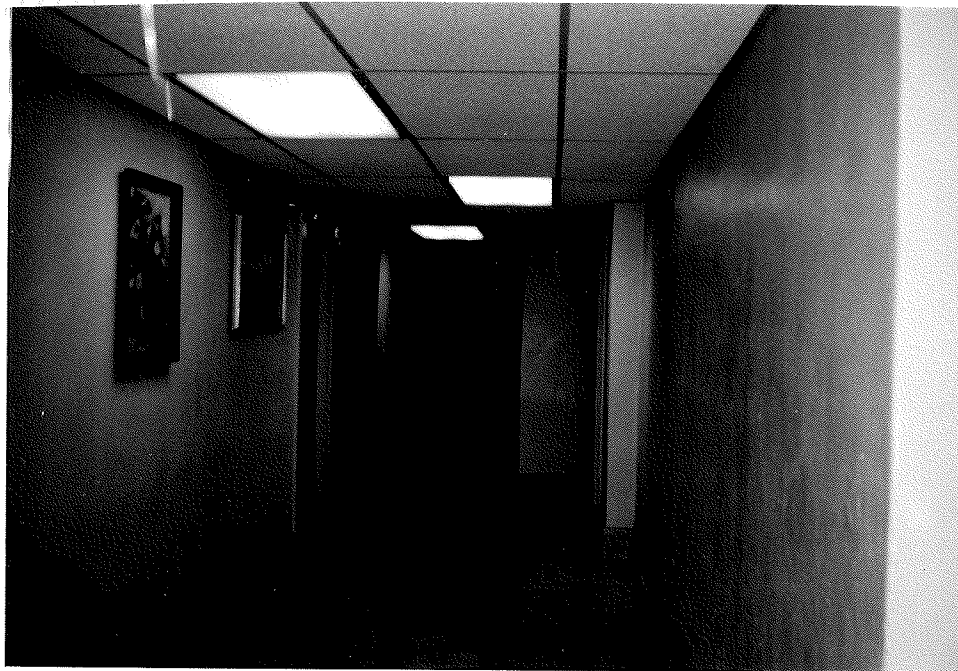
35 View to the north of the basement hallway of the Del Roy Apartments. Note the door to the crawl space located at the top of the stairs.
