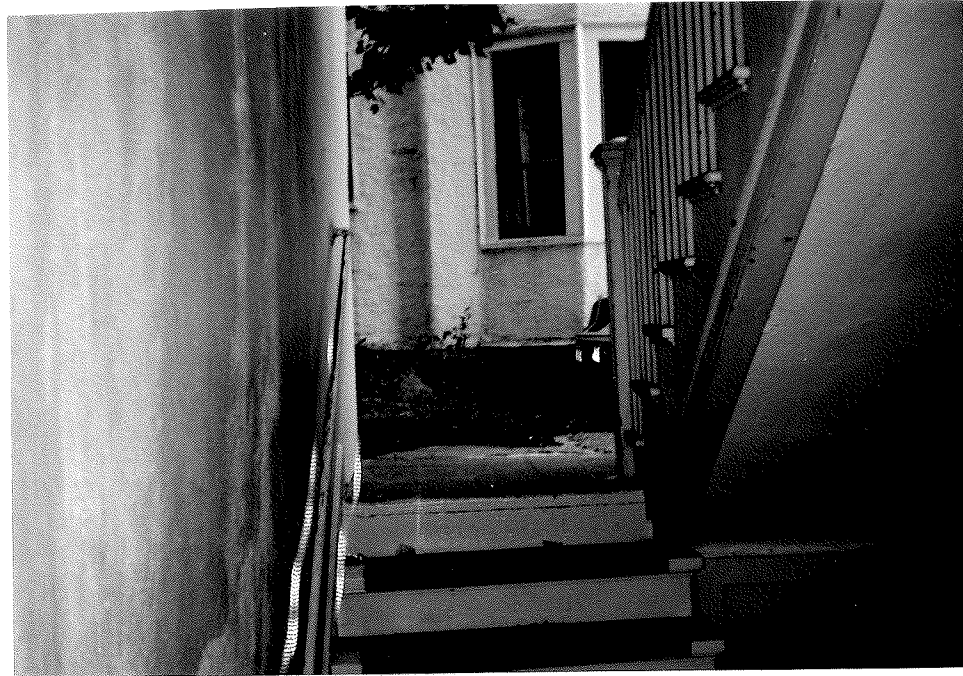
39 View to the north of the landing outside of the basement door on the south end of the Del Roy Apartments. Note the Monterey Apartments in the background.
