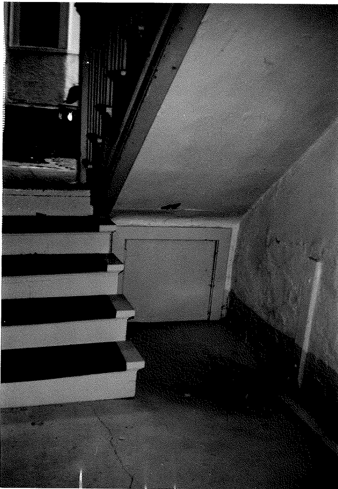
38 View to the north of the landing outside of the basement door on the south end of the Del Roy Apartments. Note the Monterey Apartments in the background.
