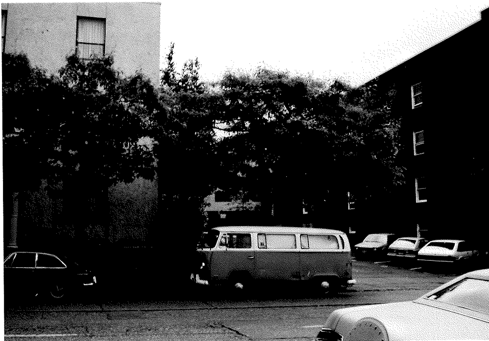
28 View to the east of the Monterey Apartments parking lot located on the south side of the building.
