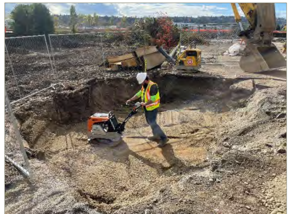
Exhibit E-9: Photos of Compaction Activities. Clockwise From Top-Left: Photo of Excavator Compacting Quarry Spalls in Area 5. View Direction is Southeast. Top-Right: Photo of Smooth-Drum Vibratory Roller in Area 1. View Direction is North. Bottom-Right: Photo of Walk-Behind Vibratory-Plate Compactor in Area 6. View Direction is Southwest. Bottom-Left: Photo of Nuclear Densometer in Area 1.
