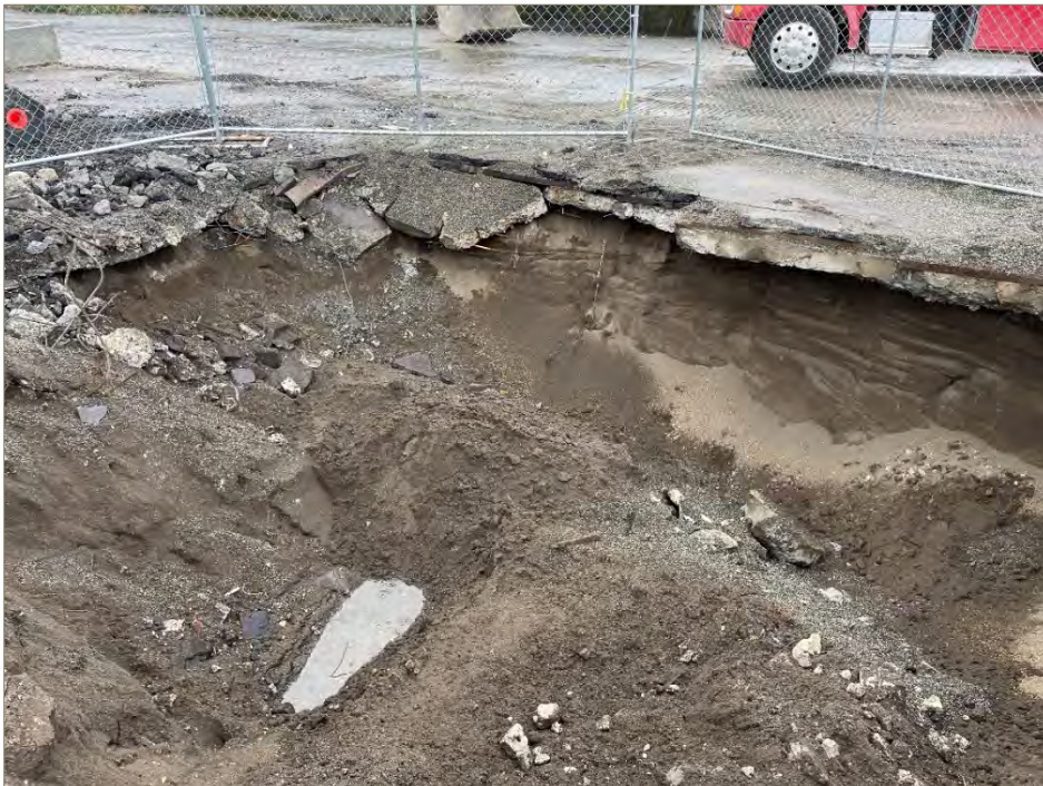
Exhibit A-24: Area 7 – View of the South Sidewall Final Extent. Photo taken on October 6, 2021. View direction is south. Groundwater was observed in the excavation bottom.
