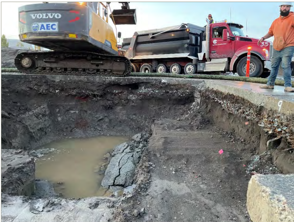
Exhibit A-8: Area 2 – View of the Southwest Portion Final Extent of the Excavation. Pink flags are sample locations. Photo taken on November 3, 2021. View direction is south. Water in the excavation is pooled rainwater and was removed prior to backfilling.
