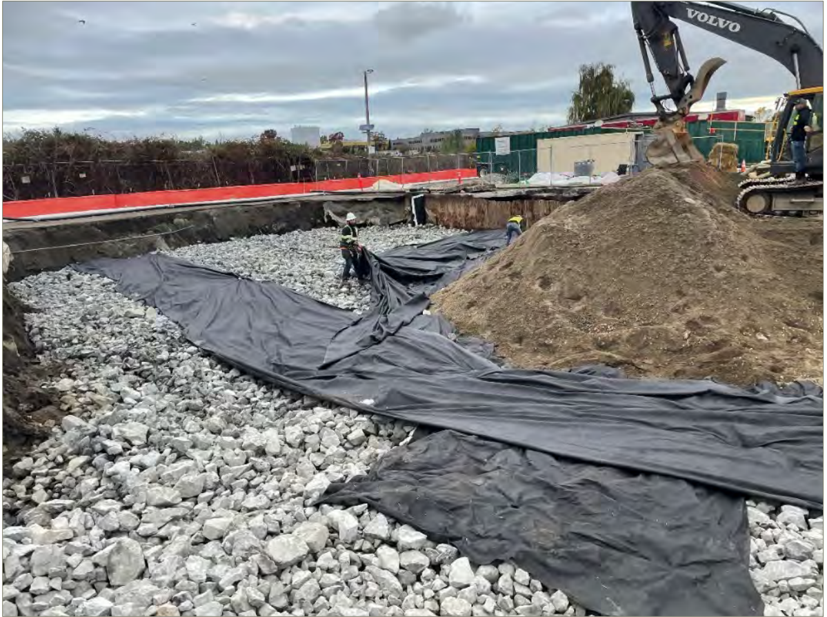
Exhibit E-7: Photo of Quarry Spalls Overlain by Geotextile Overlain by Gravel Borrow at Area 5. View Direction is Northwest.
