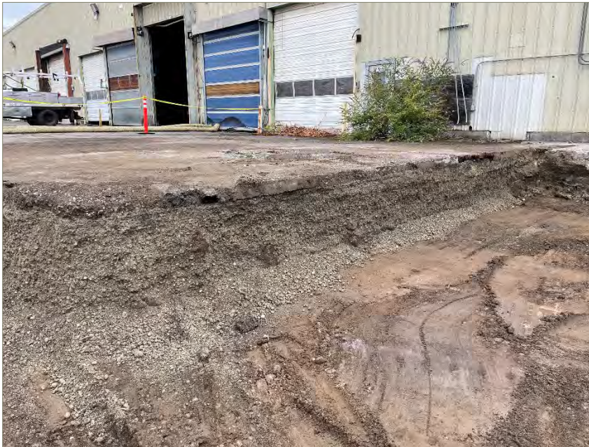
Exhibit 5-2: Photo of the Northeast Sidewall of Area 2 on September 20, 2021. View direction is northeast. The northeast sidewall was observed to have apparent imported backfill from the previous H4 excavation.
