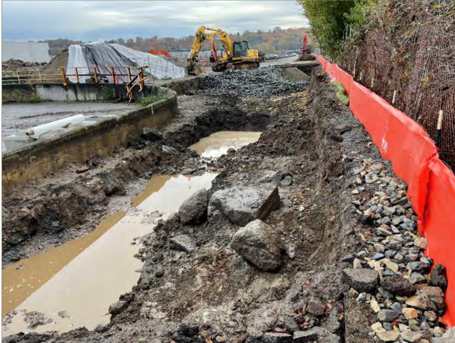
Exhibit A-12: Area 3 – View of the North Portion Final Extent of the Excavation. Photo taken on November 3, 2021. View direction is east. Water in the excavation is pooled rainwater that was removed prior to backfilling. Large rocks are part of the shoreline berm. Placement of backfill is occurring in the background.
