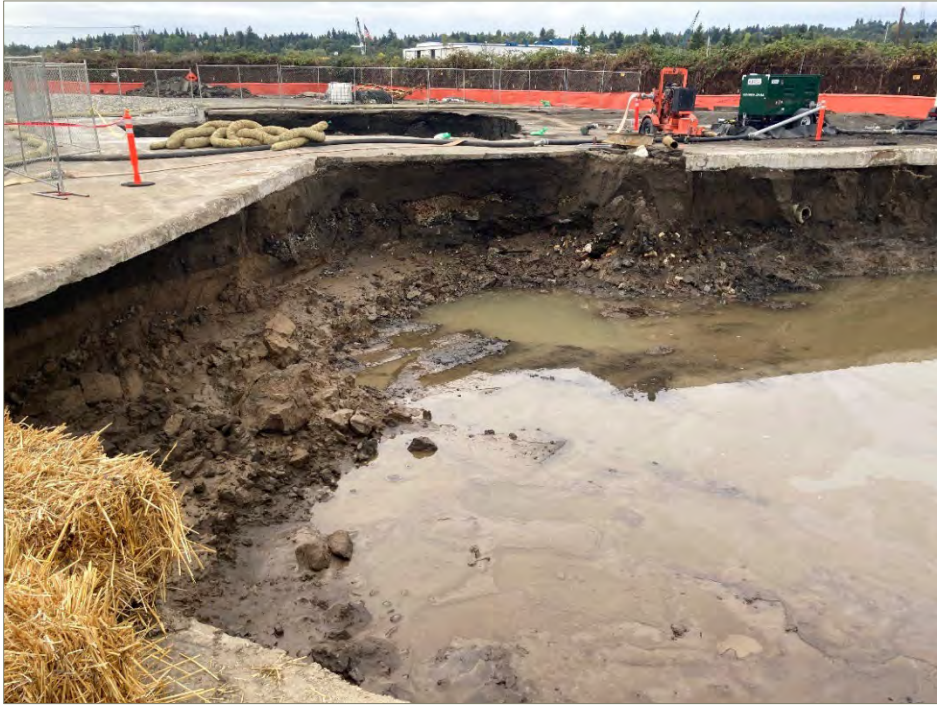
Exhibit A-17: Area 5 – View of the Southwest Portion of the Excavation. Photo taken on September 29, 2021. View direction is south. Water in the excavation is groundwater and was later removed and treated when the excavation was expanded.
