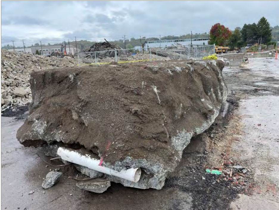
Exhibit A-22: Area 7 – View of the Concrete Vault (Upside Down) that was Removed from the Excavation. Photo taken on October 6, 2021.
