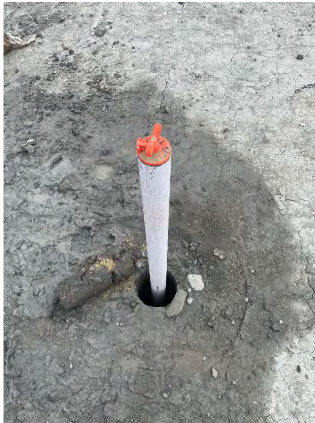
Figure 22: Completed Screen Well
