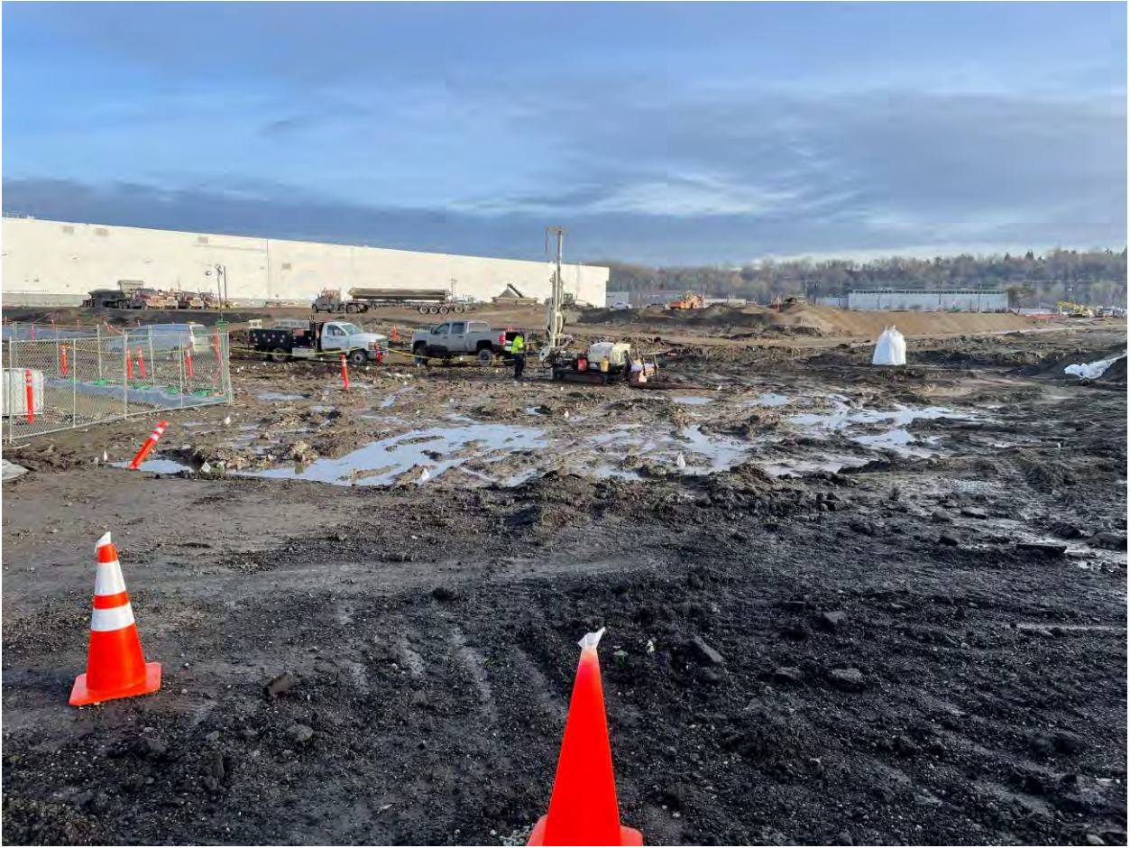
Figure 24. Area 4 drilling area overview
