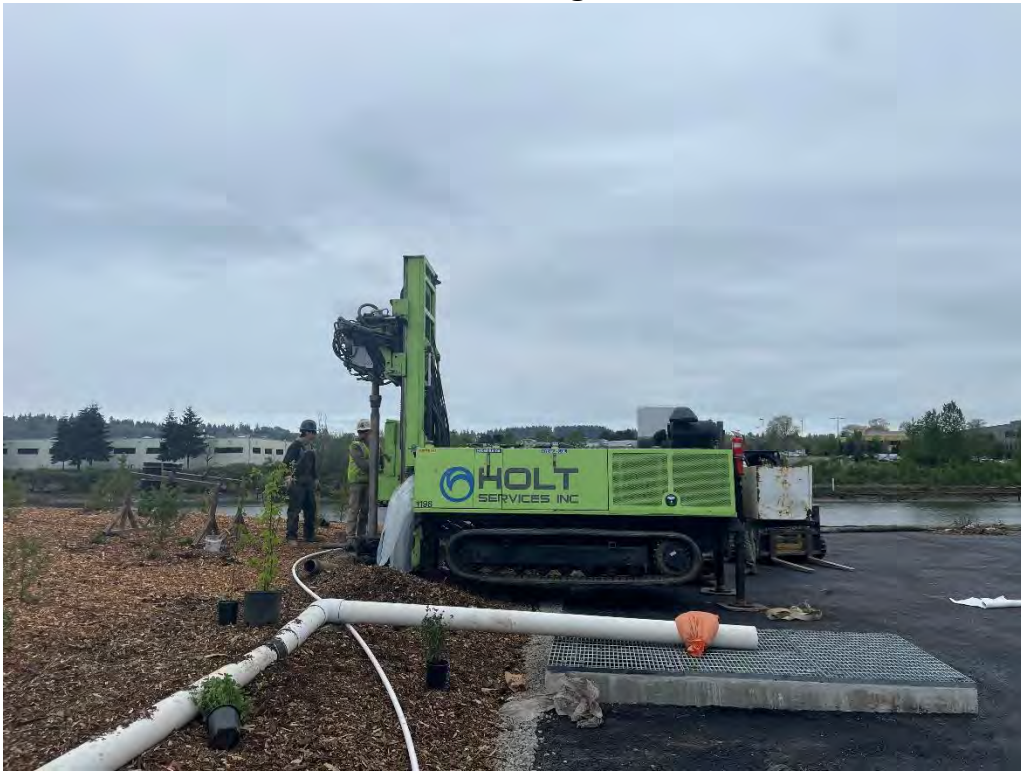
Figure 1: MW-44A(R) at start of drilling, facing W
