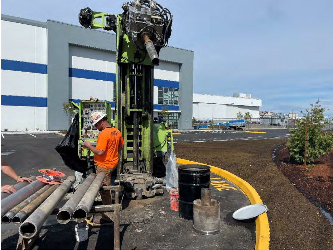
Figure 89: MW-1A(R) end drilling, facing NW
