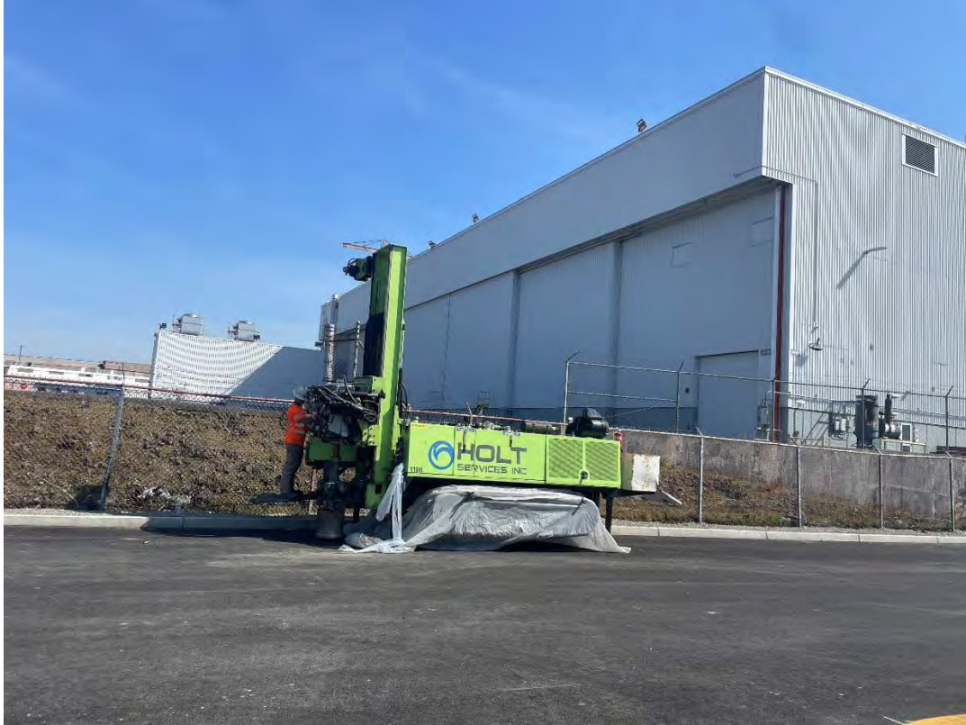
Figure 19: MW-32A(R) start of drilling, facing N
