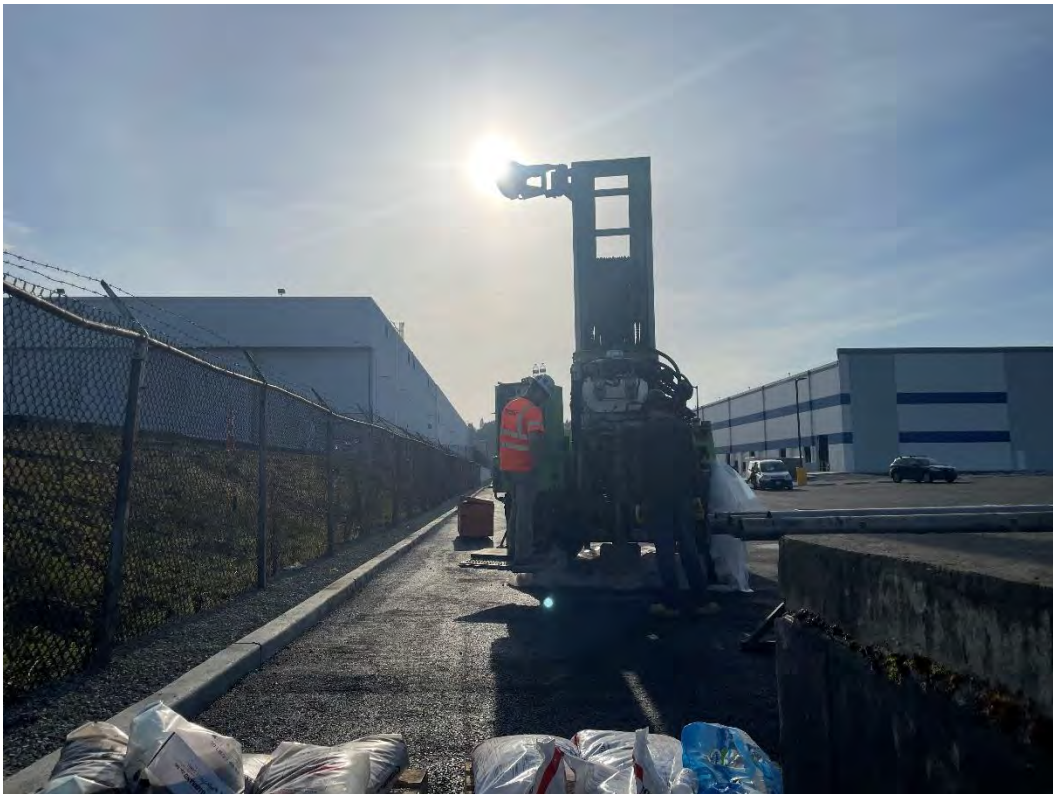
Figure 12: MW-25A(R) at start of drilling, facing E
