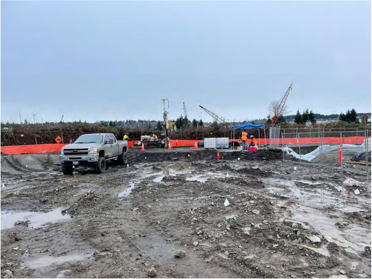
Figure 6. Area 4 drilling area overview
