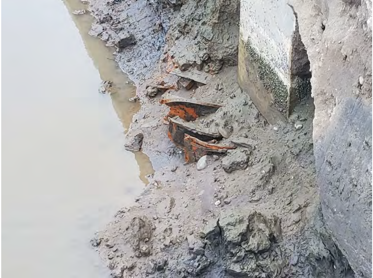
Figure 2. Concrete, possible bank armor for river, found under asphalt ramp
