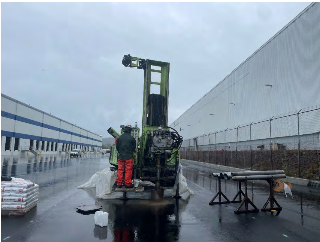
Figure 78: MW-16A(R) start drilling, facing W
