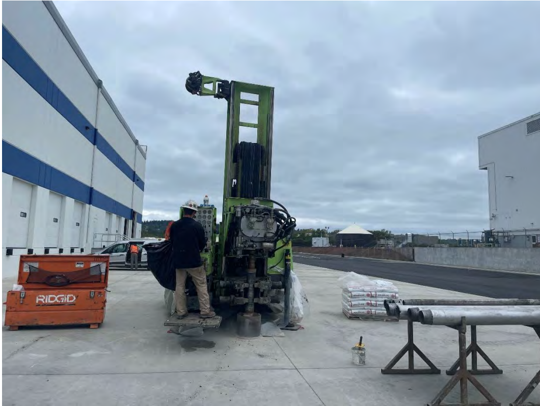
Figure 61: MW-18A(R) start drilling, facing W
