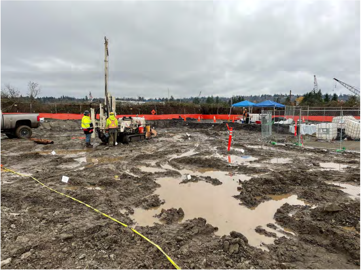
Figure 15. Area 4 drilling area overview
