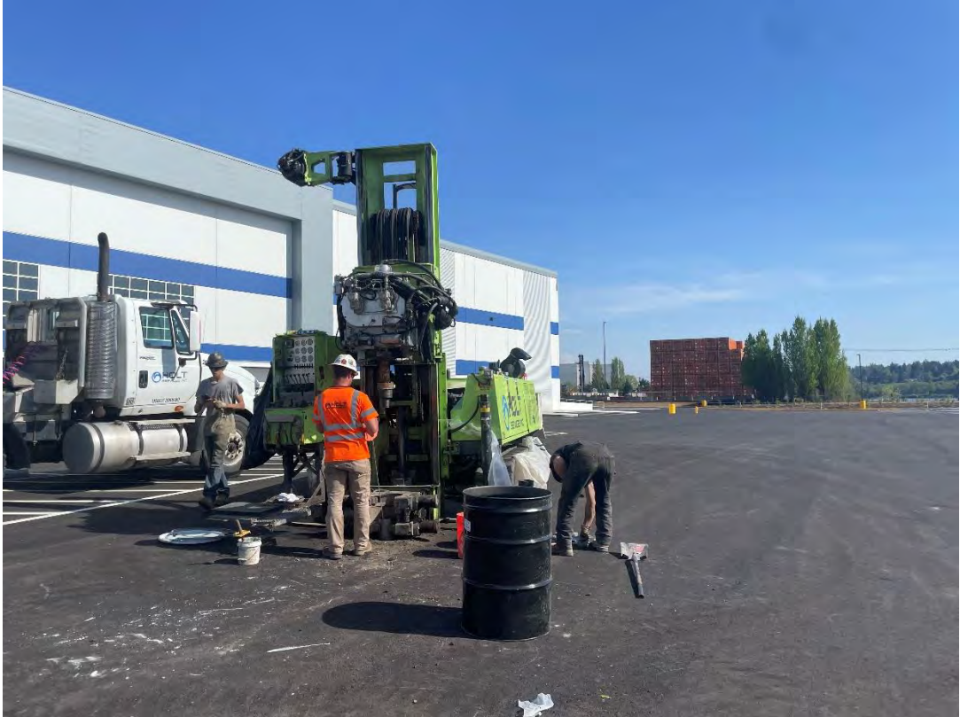
Figure 38: MW-47A(R) end of drilling, facing SE
