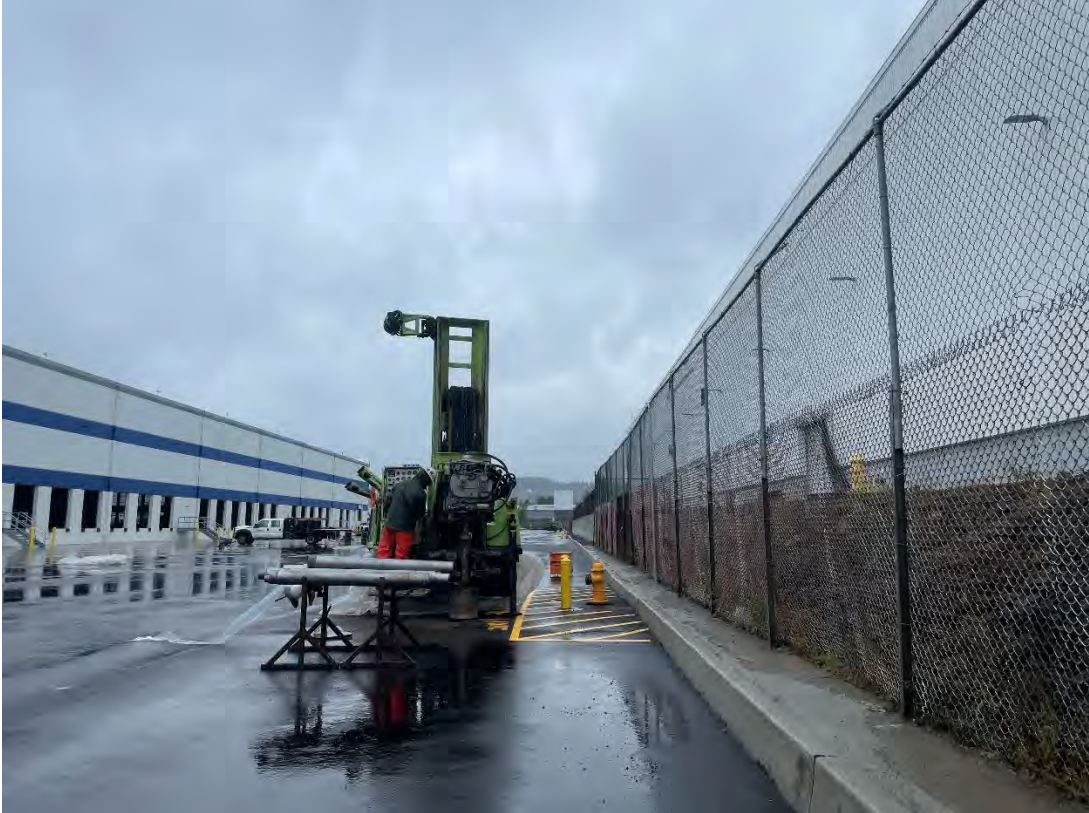
Figure 72: MW-34A(R) start of drilling, facing W
