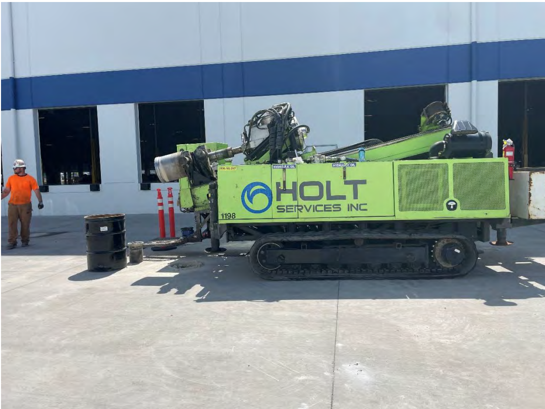
Figure 94: MW-18A(R) Pavement redrilling end, facing S
