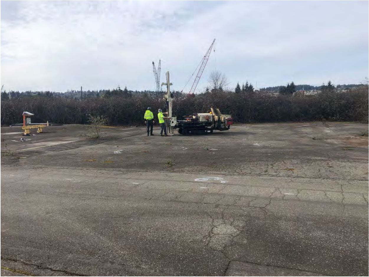
Figure 5. Drilling being done in Area 5-7, 11:58am
