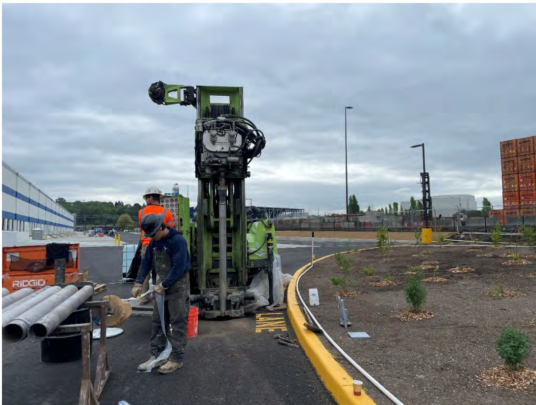
Figure 50: MW-41A(R) start of drilling, facing N
