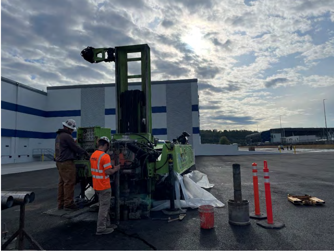
Figure 45: MW-12A(R) Start of drilling, (continued 5/8/2023), facing E
