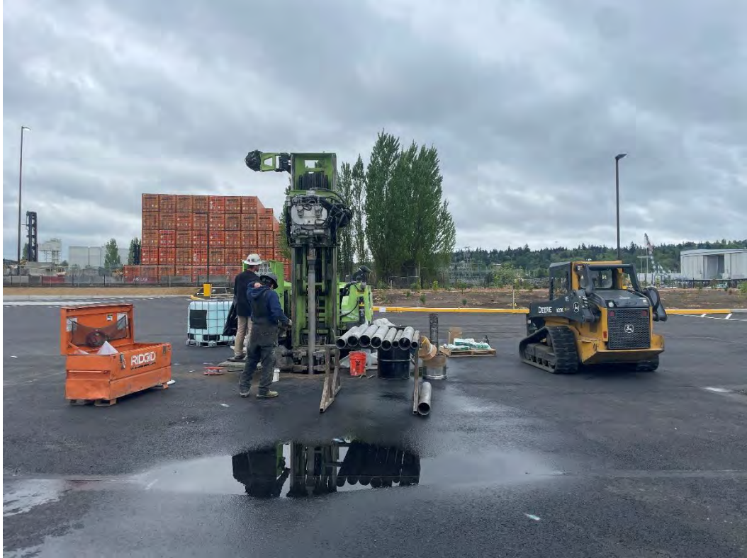
Figure 39: MW-12A(R) start of drilling, facing S
