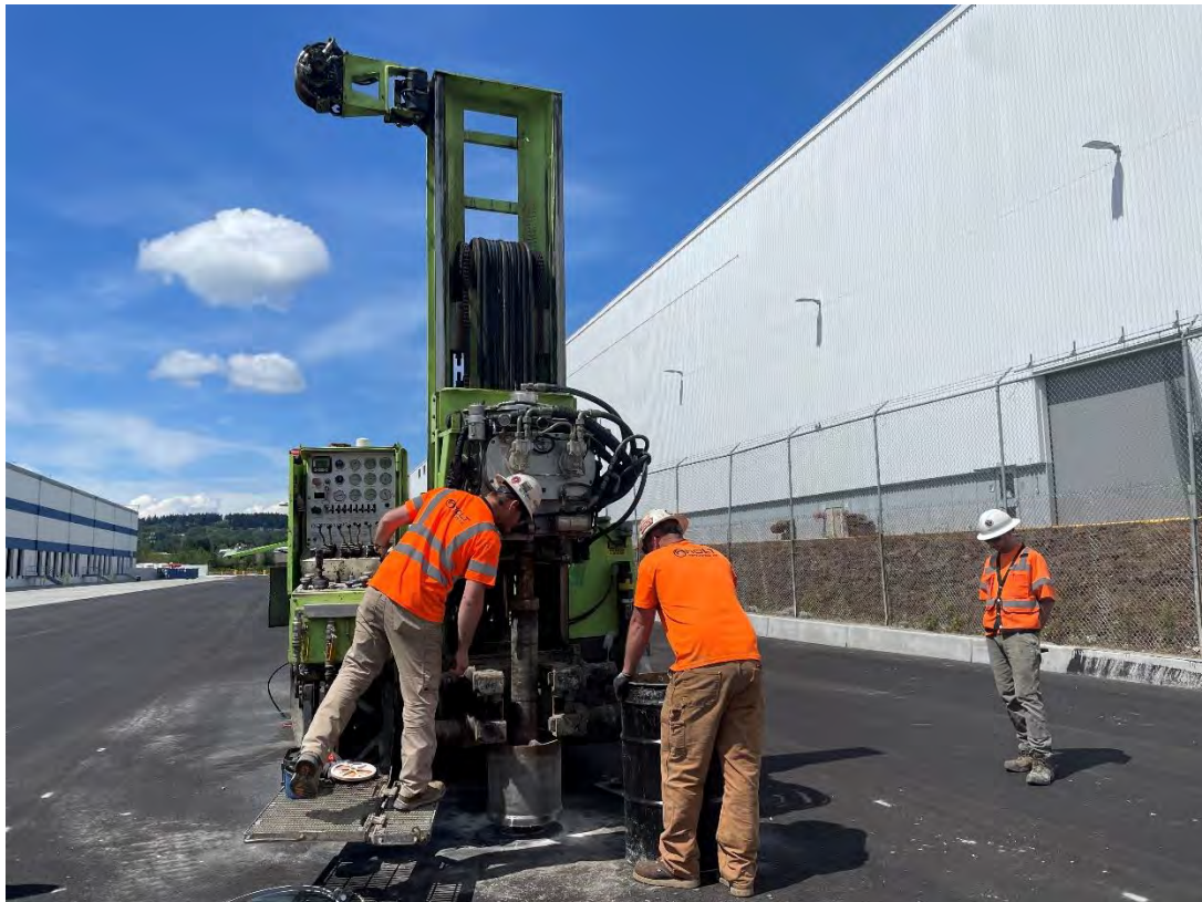
Figure 92: MW-16A(R) Pavement redrilling end, facing W
