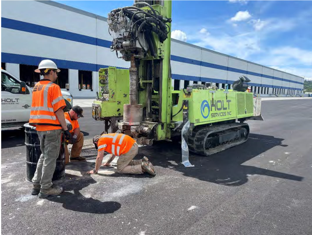
Figure 91: MW-16A(R) pavement redrilling start, facing NW
