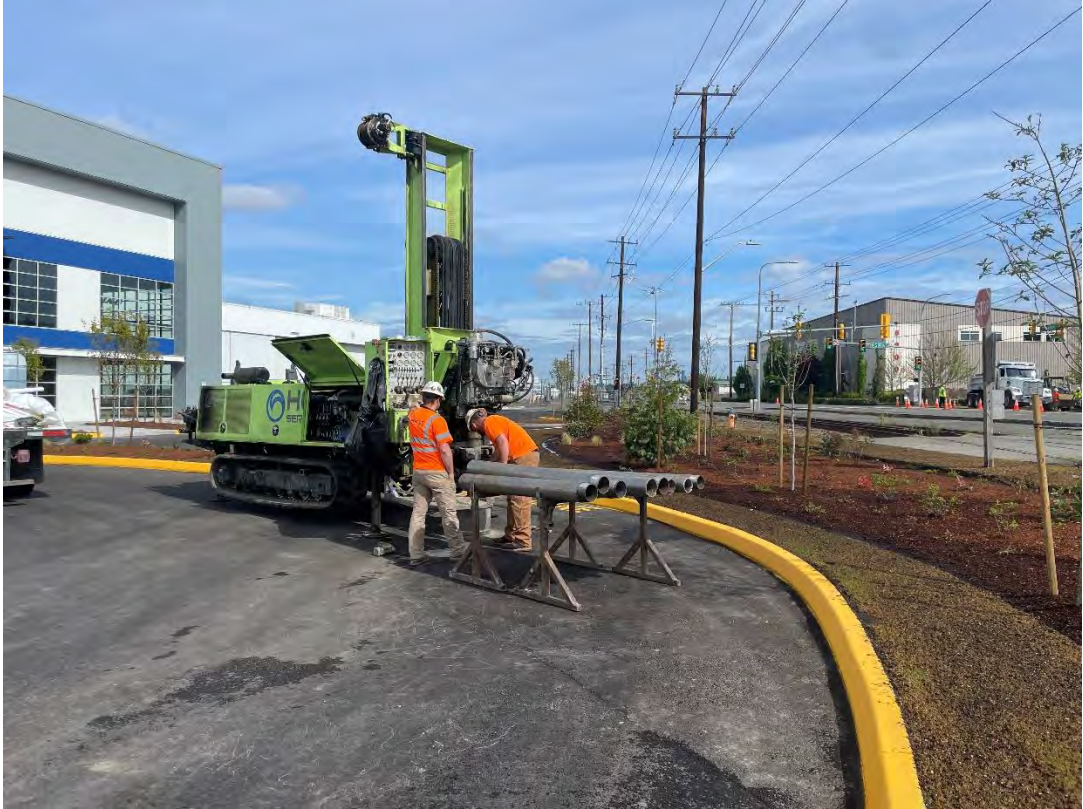
Figure 85: MW-1A(R) start drilling, facing N
