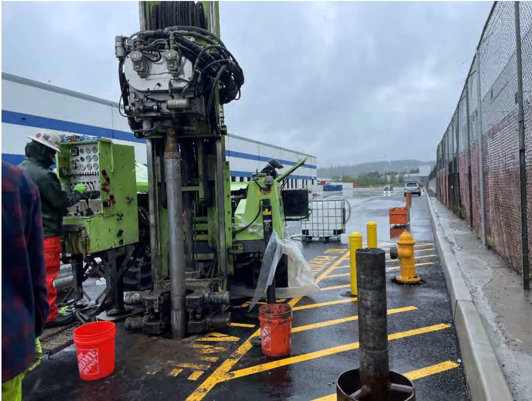
Figure 77: MW-34A(R) end of drilling, facing SW
