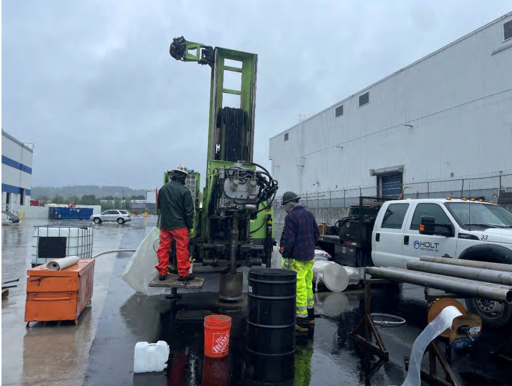
Figure 67: MW-14A(R) start drilling, facing W
