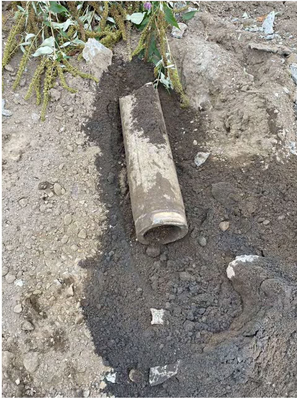
Figure 6. Asbestos pipe from Area 4
