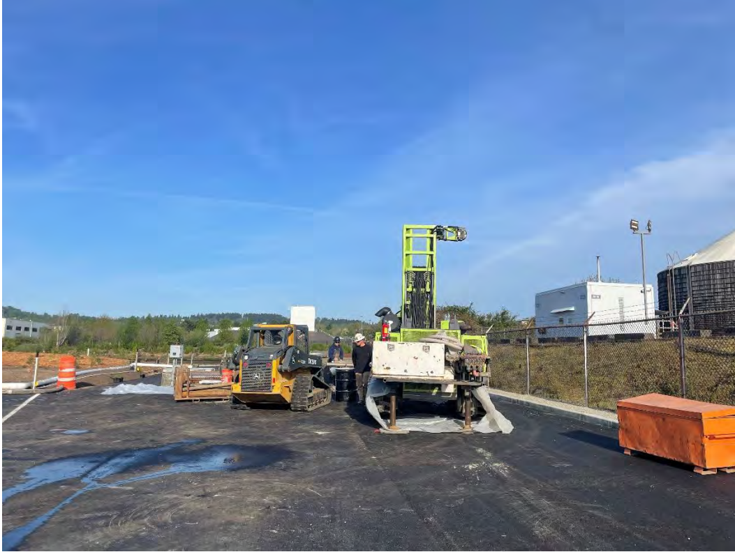
Figure 11: MW-7A(R) end of drilling, facing W
