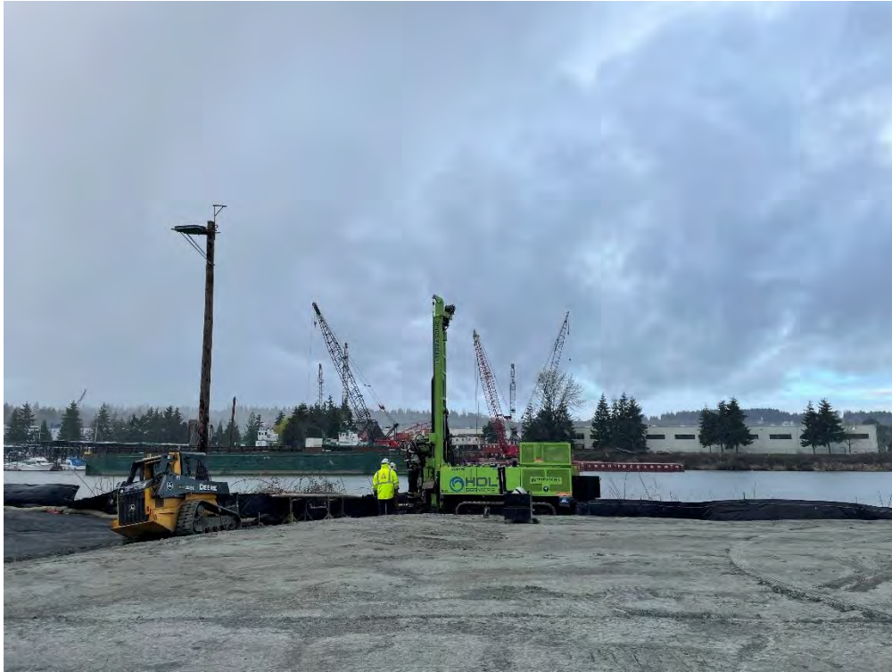
Figure 1: MW-43A(R) Overview at Start of Drilling, Facing W
