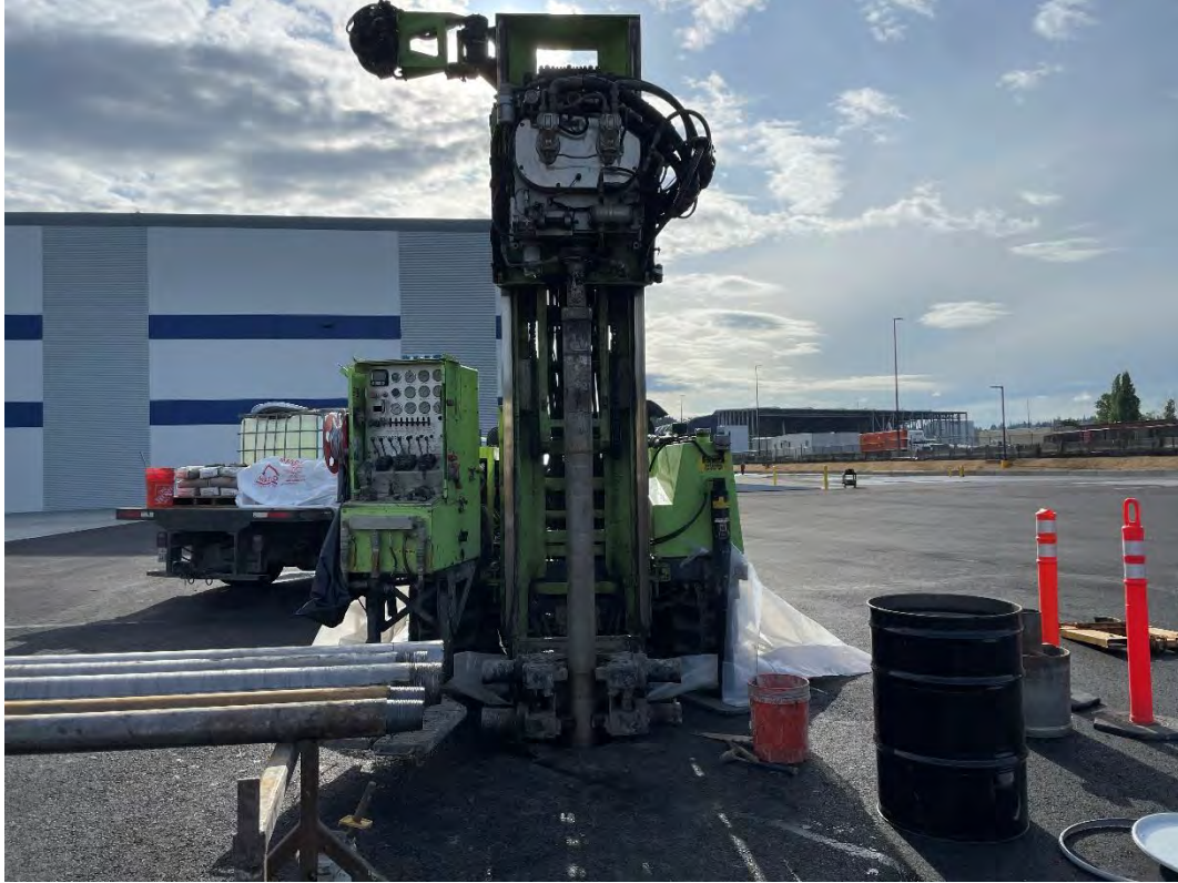
Figure 49: MW-12A(R) end of drilling
