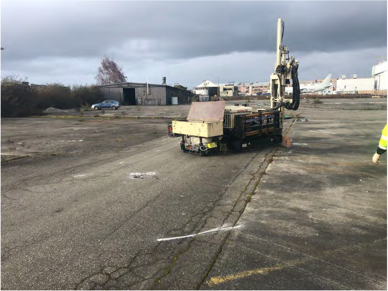
Figure 8. Drill rig being set up in area 5 3:35pm
