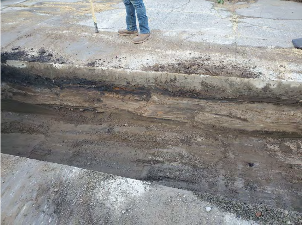
Figure 1. Area 2 side wall
