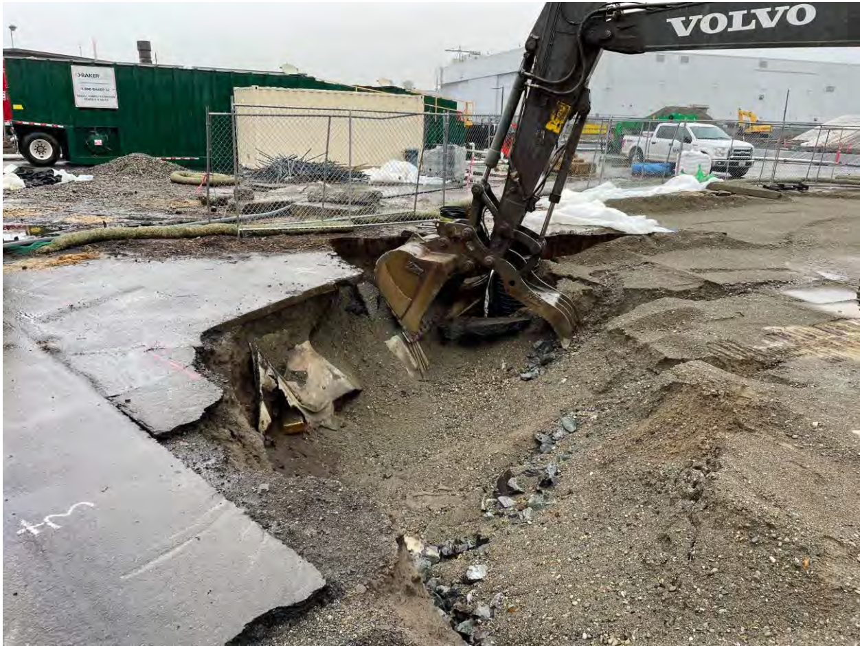
Figure 8. Area 5 Concrete in fill layer.
