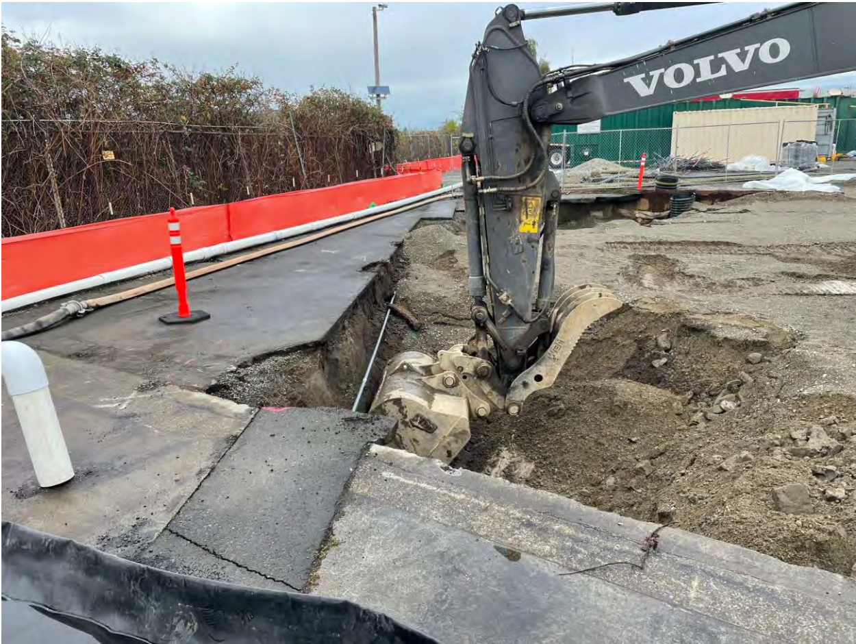
Figure 7. Area 5 Brick and concrete
