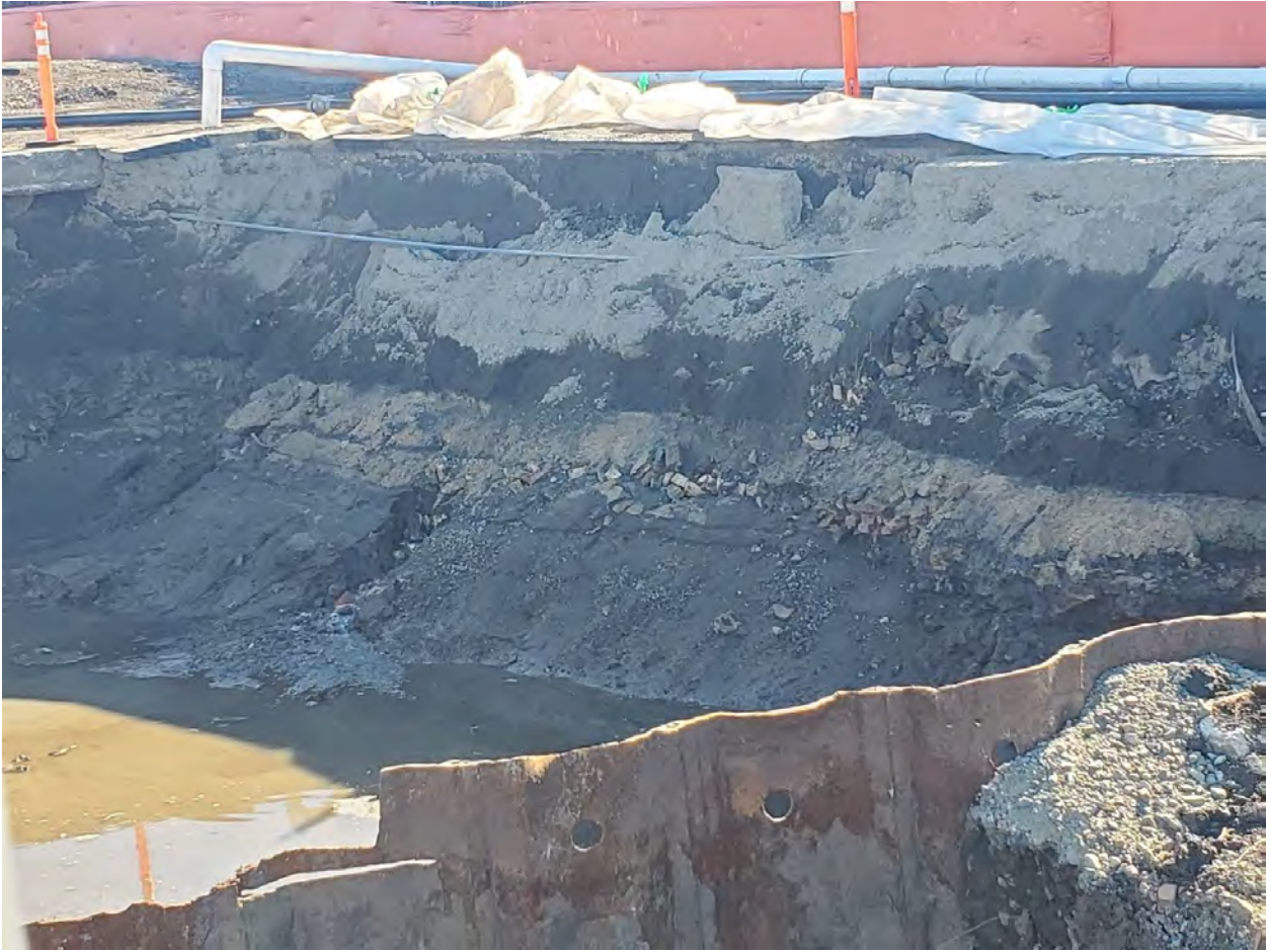
Figure 3. Brick visible in side wall in Area 5
