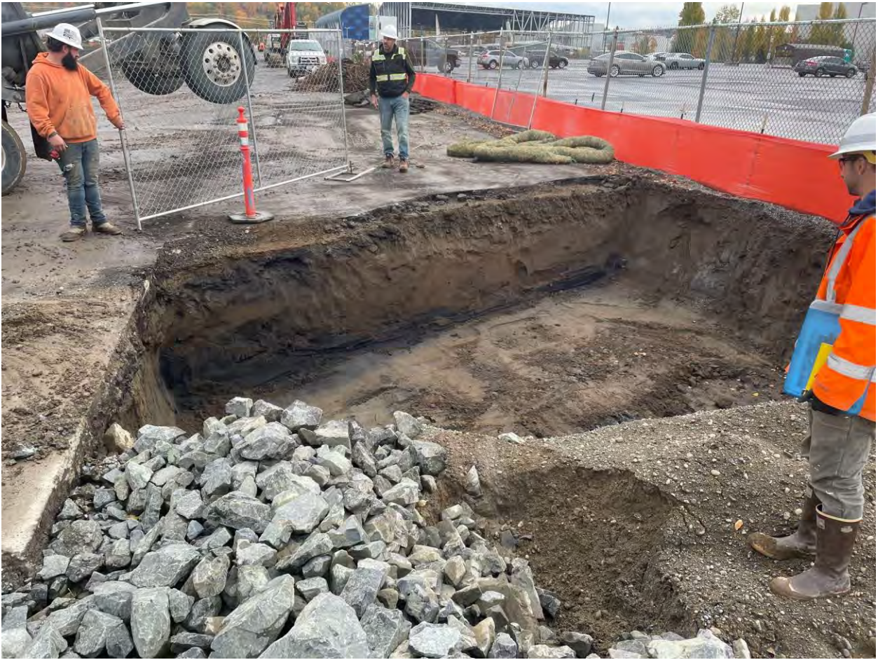
Figure 6. Area 3 eastern end overview
