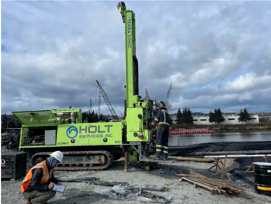
Figure 11: MW-30A(R) Overview at End of Drilling, Facing W
