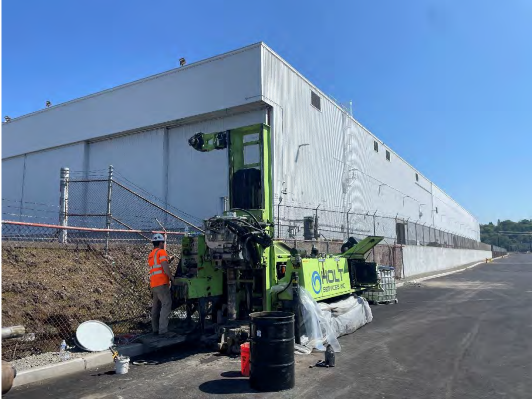
Figure 25: MW-32A(R) end of drilling, facing SE
