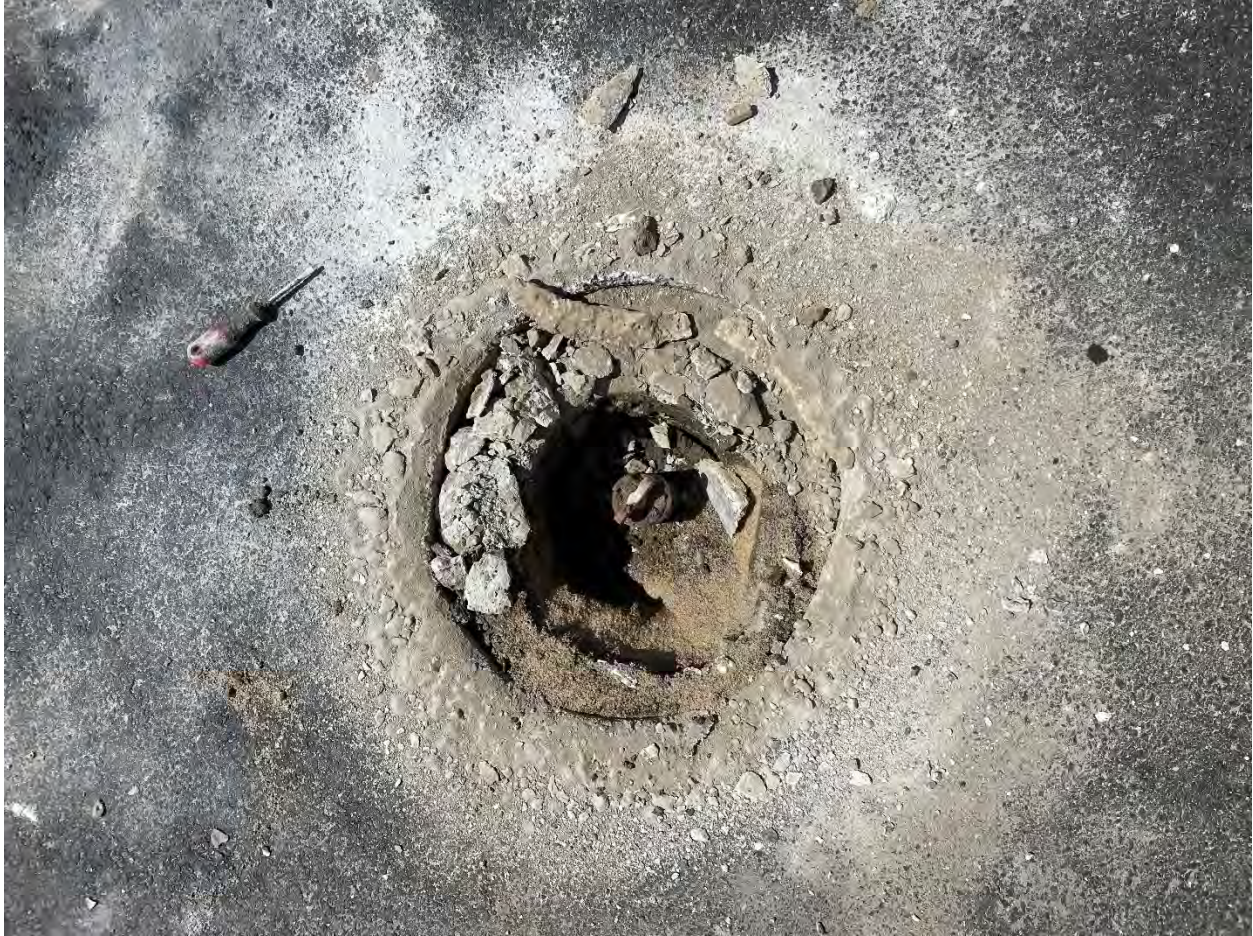
Figure 95: Completed redrilled pavement for well modification
