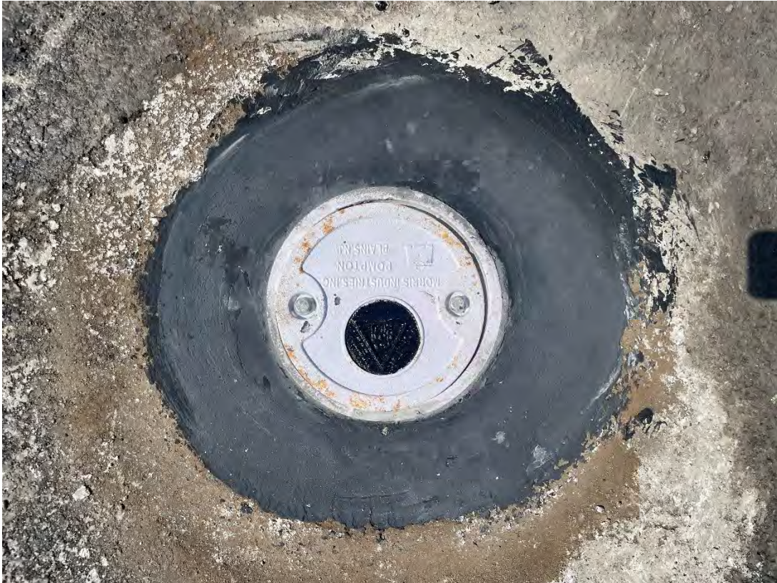
Figure 90: Completed Well Modification
