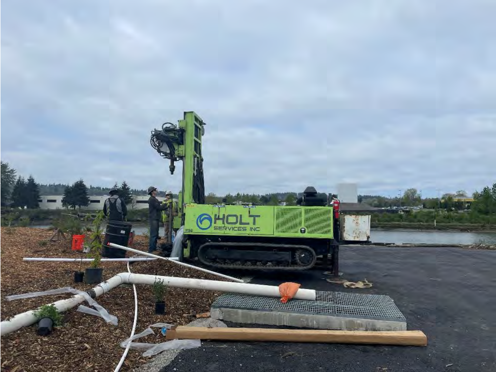
Figure 6: MW-44A(R) at end of drilling, facing W
