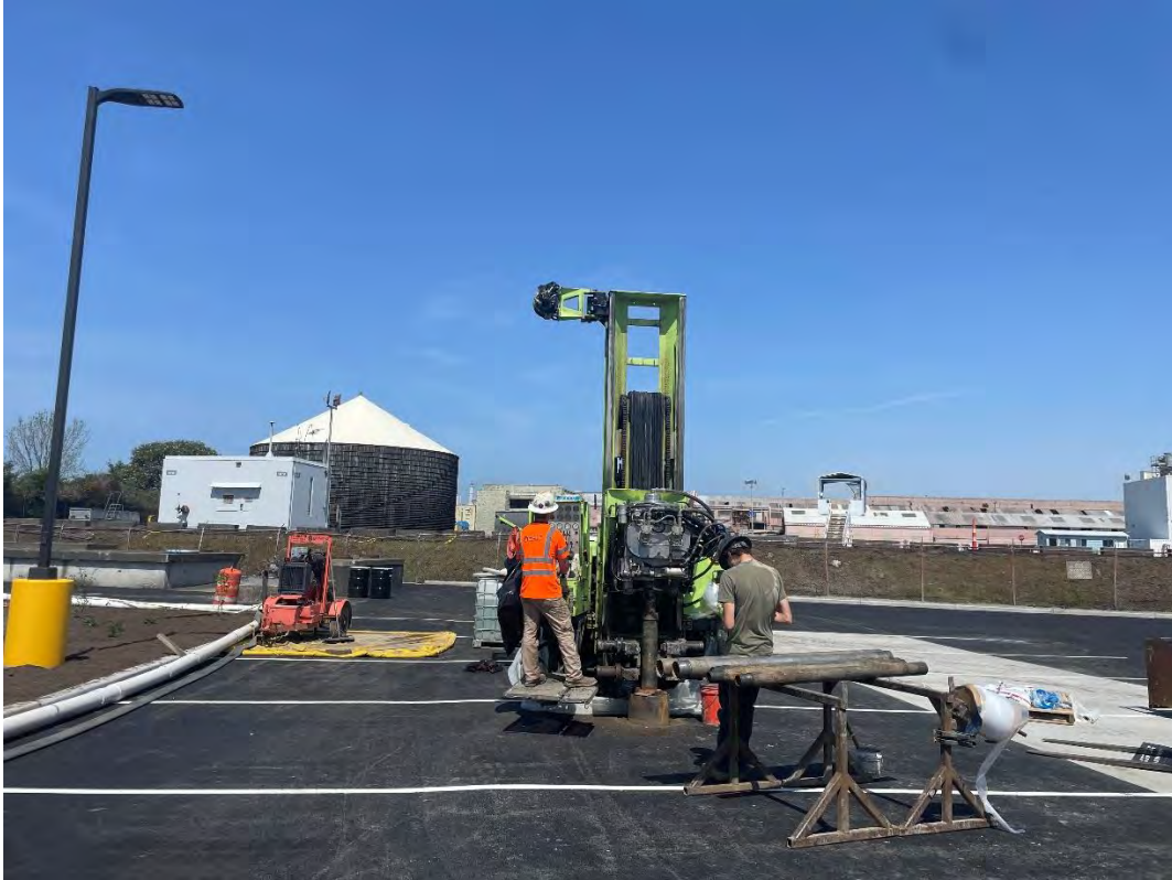
Figure 7: MW-7A(R) at start of drilling, facing N
