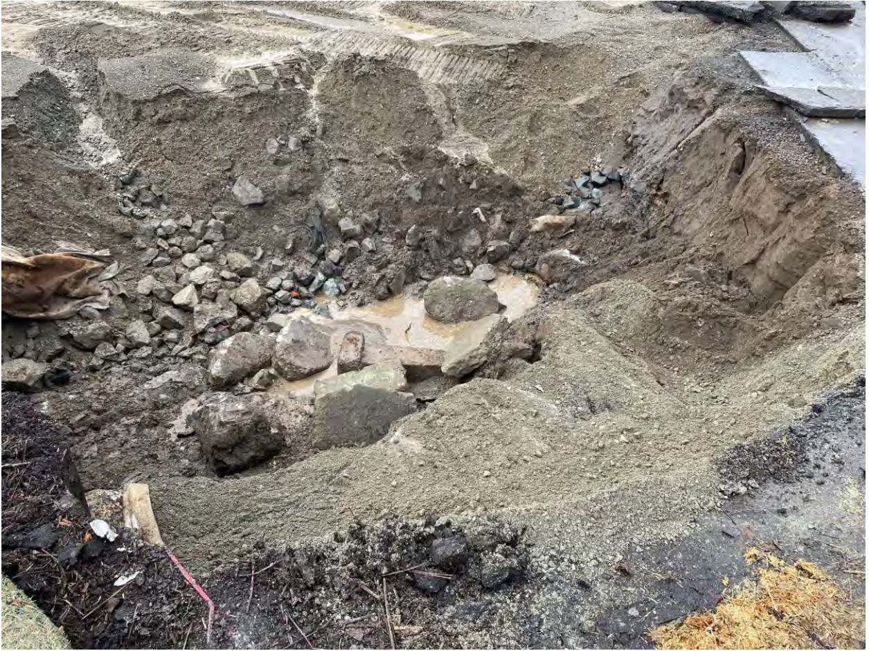
Figure 9. Area 5 More concrete in fill layer
