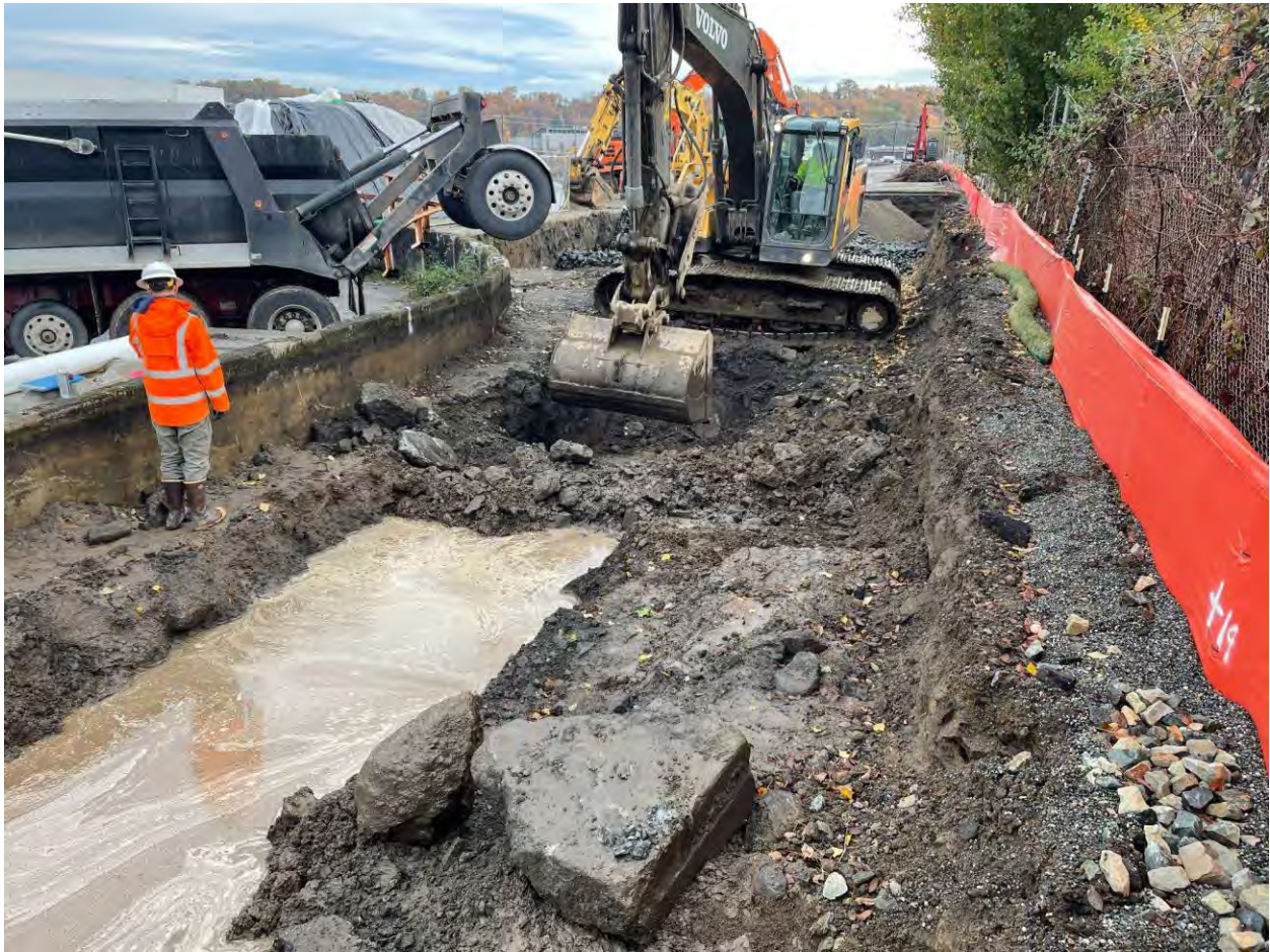
Figure 4. Area 3 western end with brick and concrete
