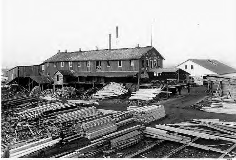
Figure 2-11. 1907 photograph of the Newell Mill in Seattle. The record notes that the site sat on the corner of S Bradford St & 7 th Ave (not within the APE) and focused on manufacturing sashes and doors (Asahel Curtis, 1907)
