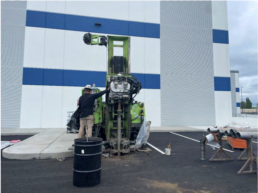
Figure 56: MW-48A(R) start of drilling, facing N
