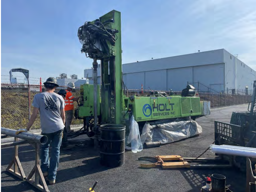
Figure 18: MW-25A(R) end of drilling, facing NE
