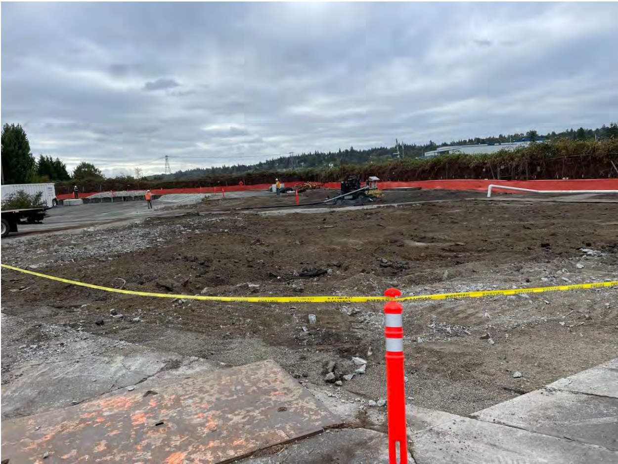
Figure 2. Area 5 prior to excavation
