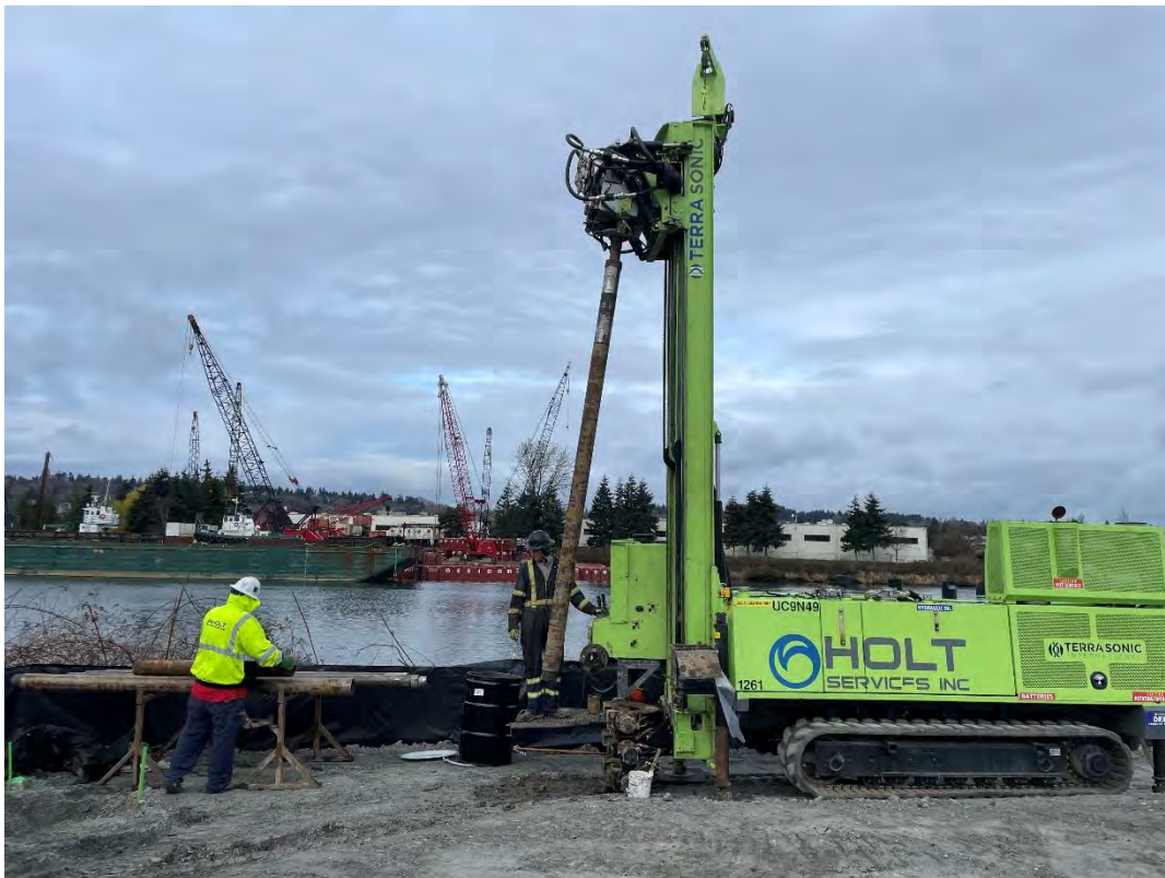
Figure 6: MW-43A(R) Overview at End of Drilling, Facing W
