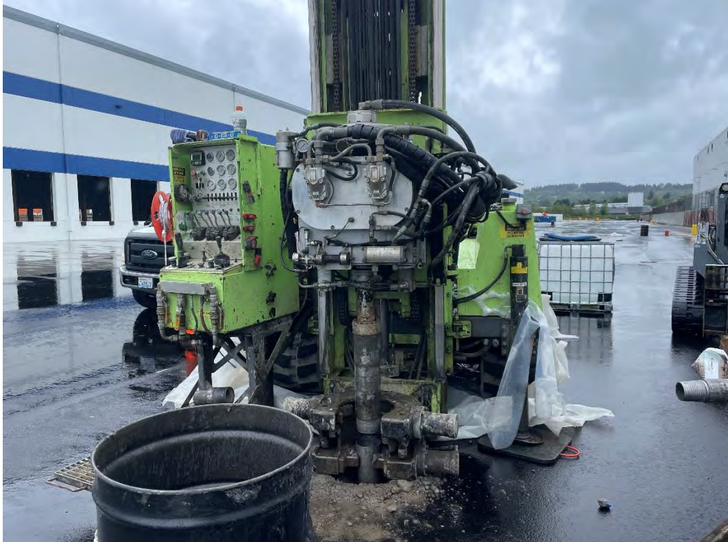
Figure 84: MW-16A(R) end drilling, facing SW
