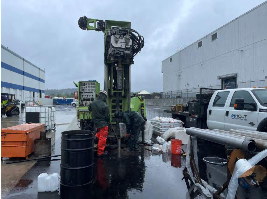
Figure 71: MW-14A(R) end of drilling, facing W
