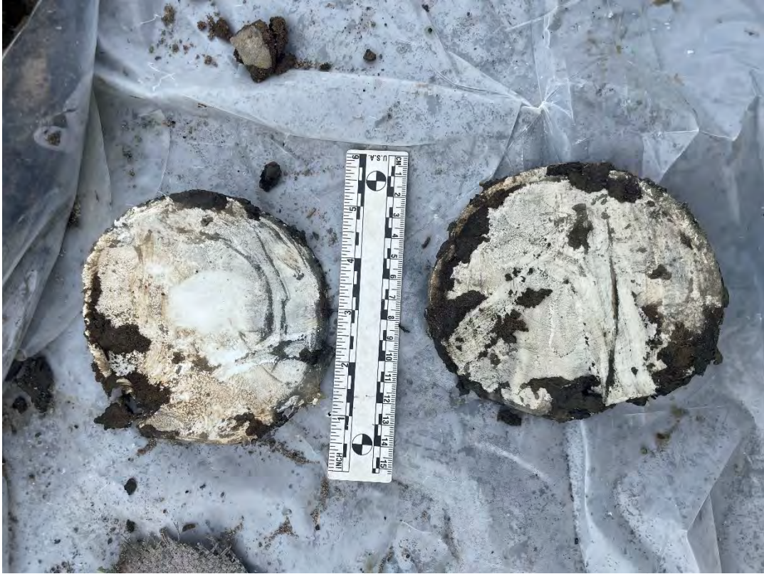
Figure 43: Unspecified PCV Weather Pipe drilled into at ~2.5-3 ft bgs
