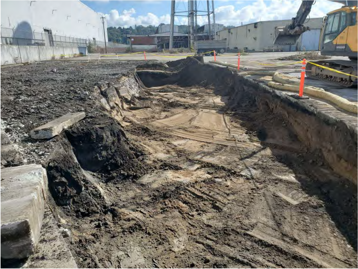
Figure 4. Partial excavation of Area 1
