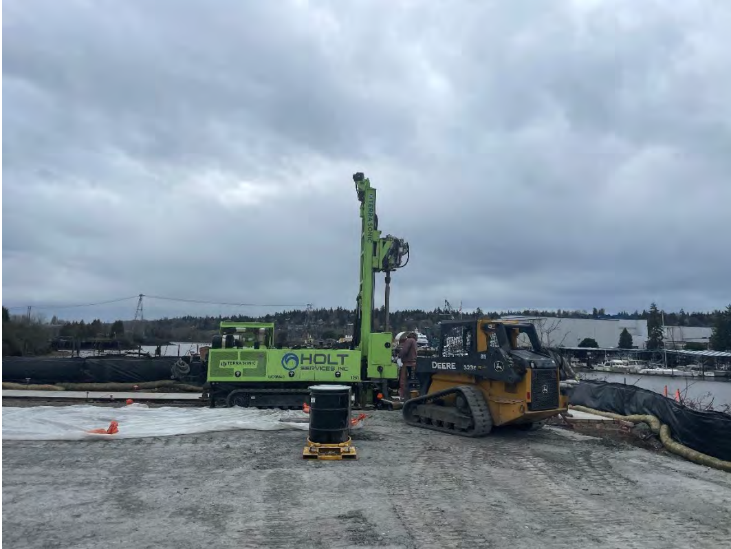
Figure 17: MW-50A Overview at Start of Drilling, Facing S
