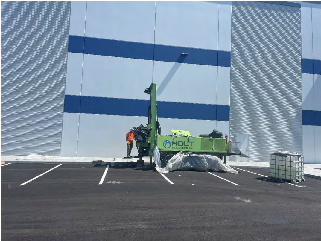
Figure 26: MW-28A(R) start of drilling, facing E
