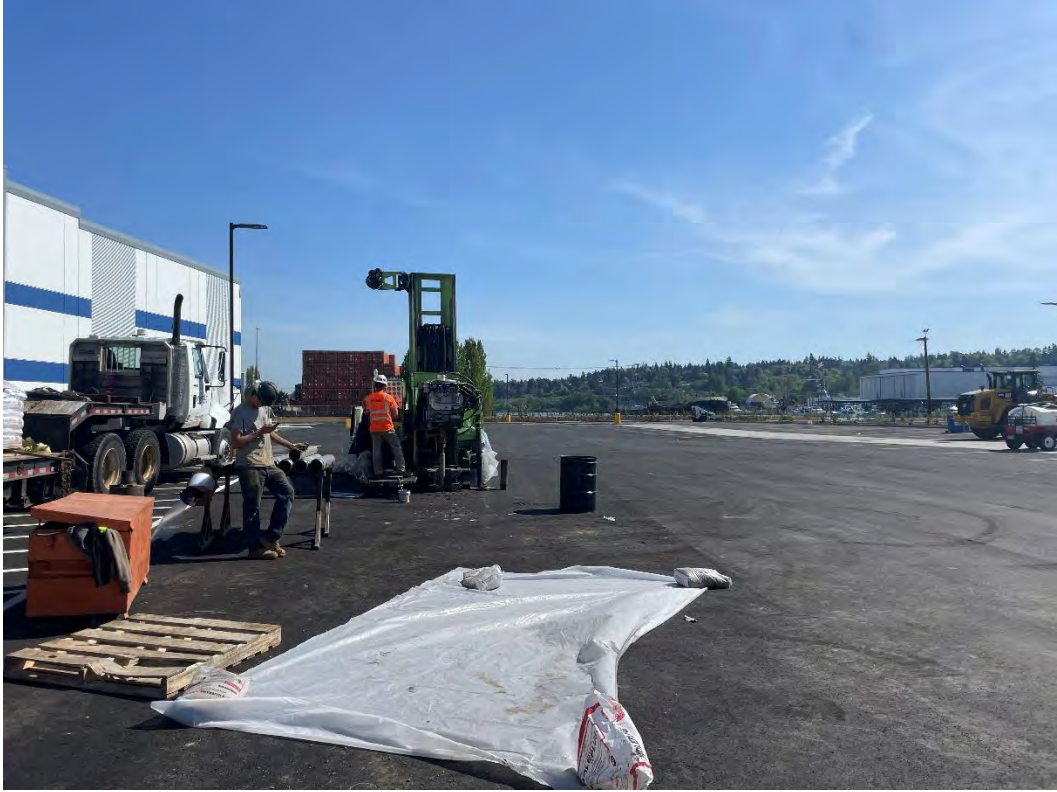
Figure 33: MW-47A(R) start of drilling, facing S
