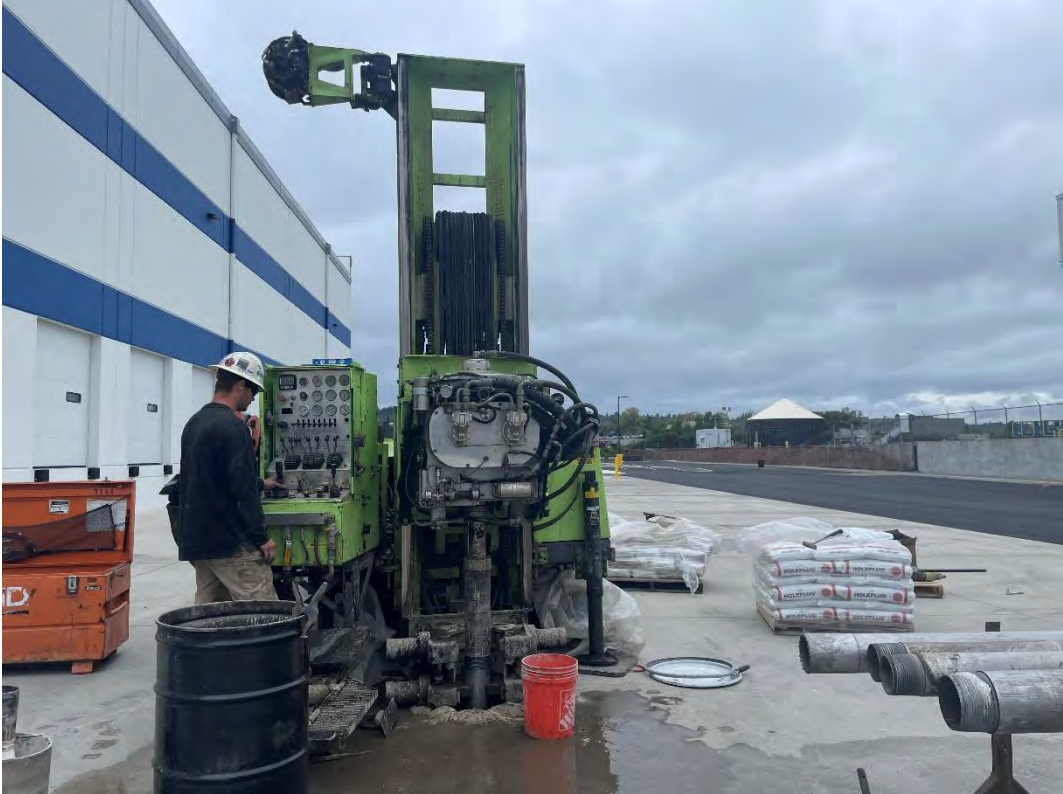
Figure 66: MW-18A(R) end drilling, facing W
