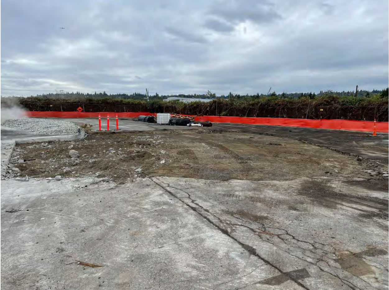
Figure 1. Area 4 prior to excavation
