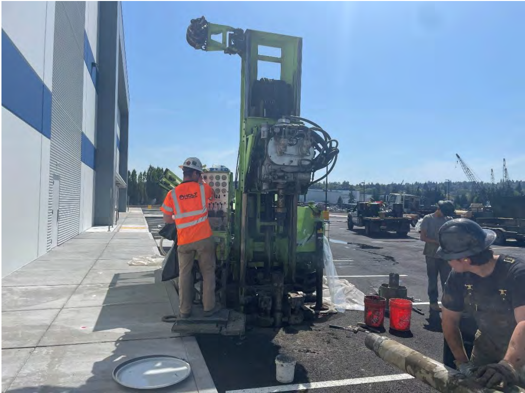
Figure 32: MW-28A(R) end of drilling, facing S
