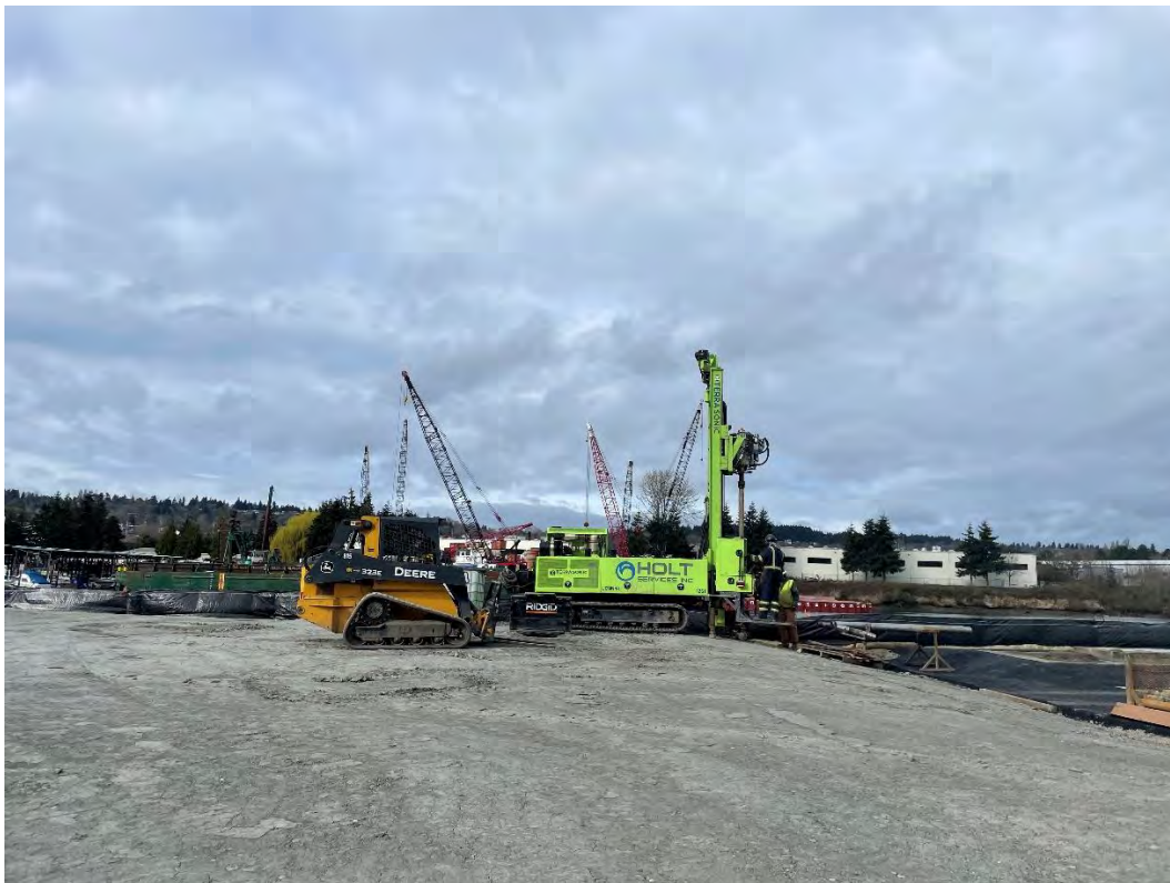
Figure 8: MW-30A(R) Overview at Start of Drilling, Facing W
