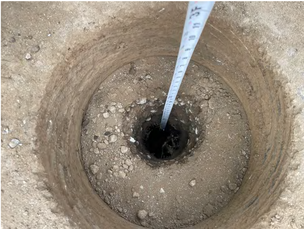
Figure 44: Drill depth that Unspecified PVC Weather Pipe was drilled into
