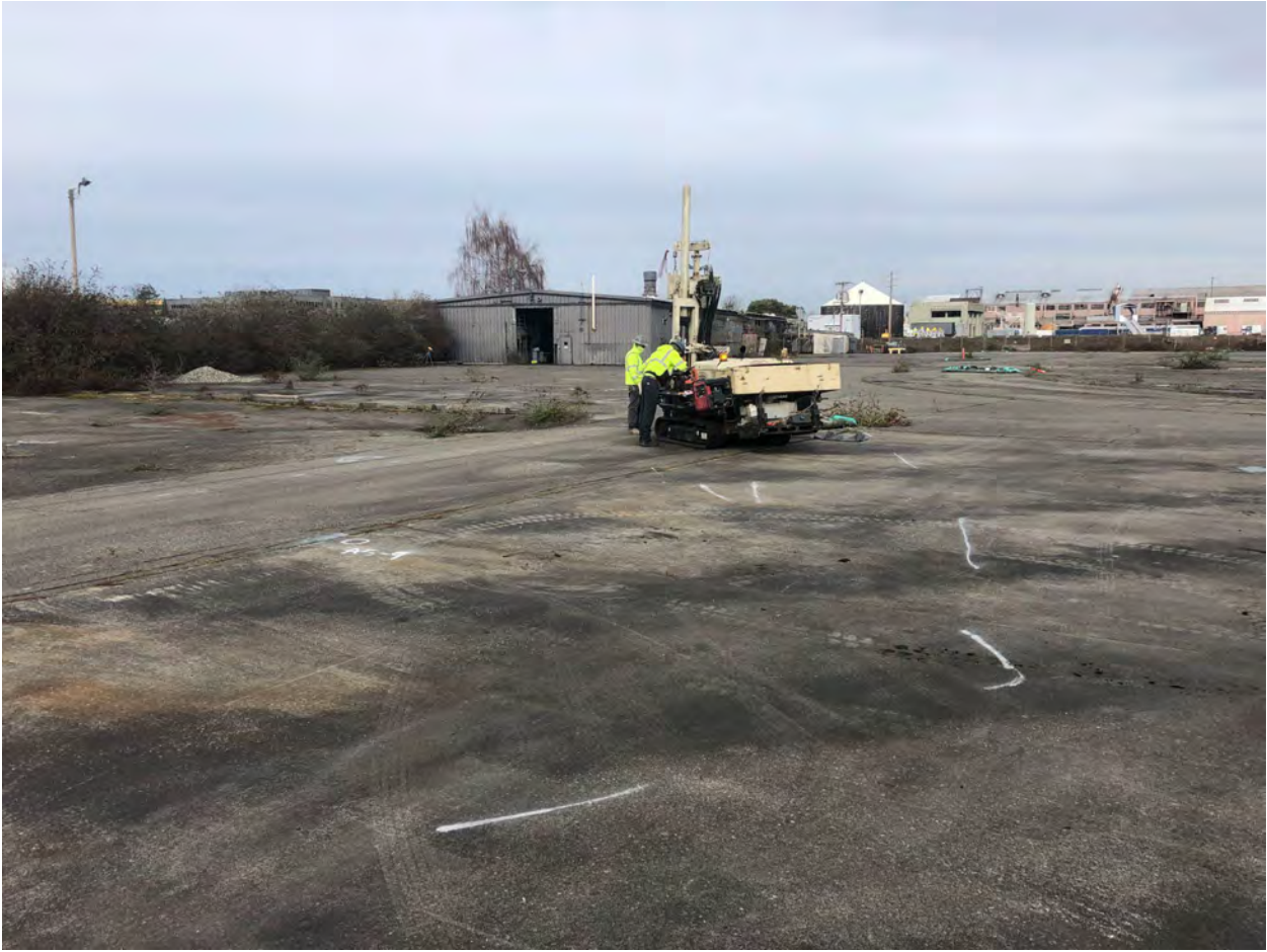
Figure 1. Drill rig being set up in Area 5-4, 10:47am
