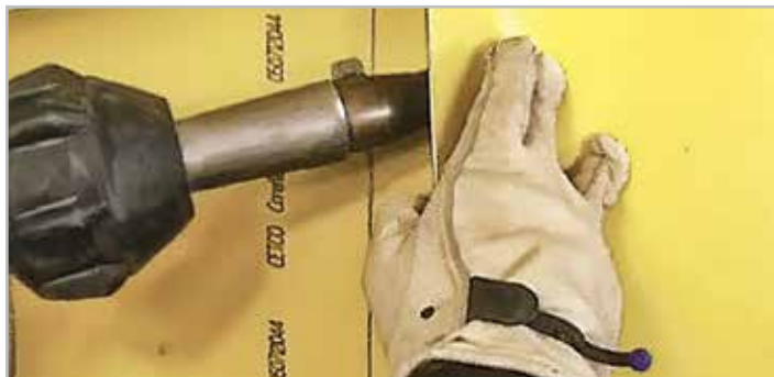
STEP 1. Tack Welding
