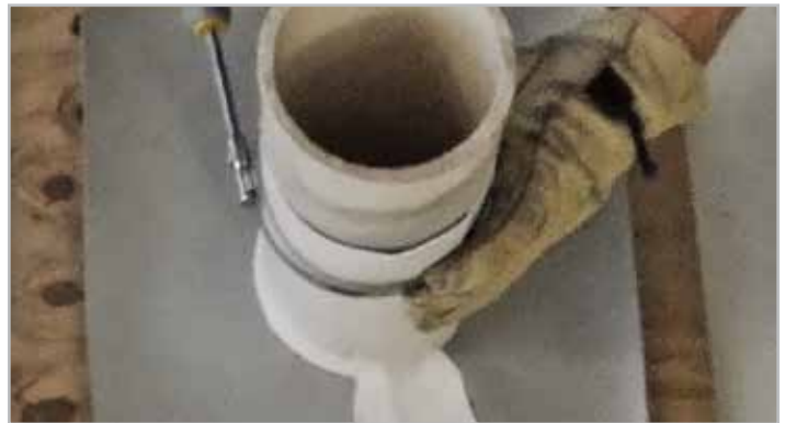
STEP 5. Install lower clamp
