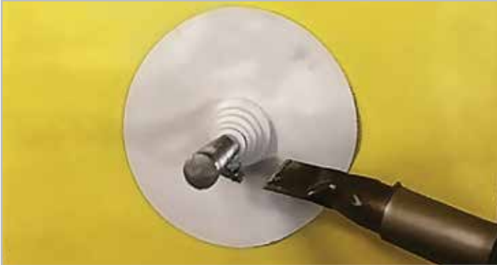
STEP 7. Hot-air applied to stepped stack
