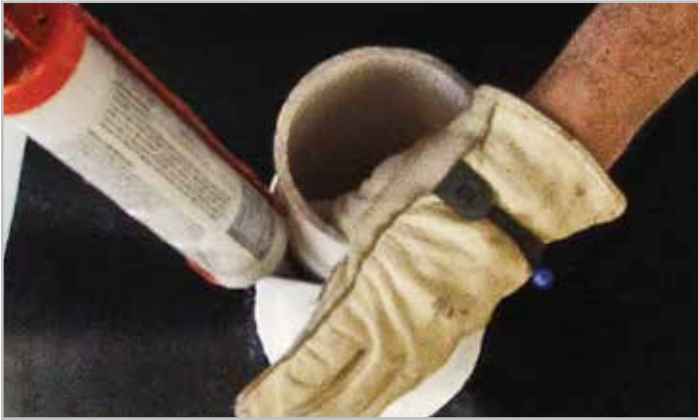
STEP 7. Install AKWASWELL bead
