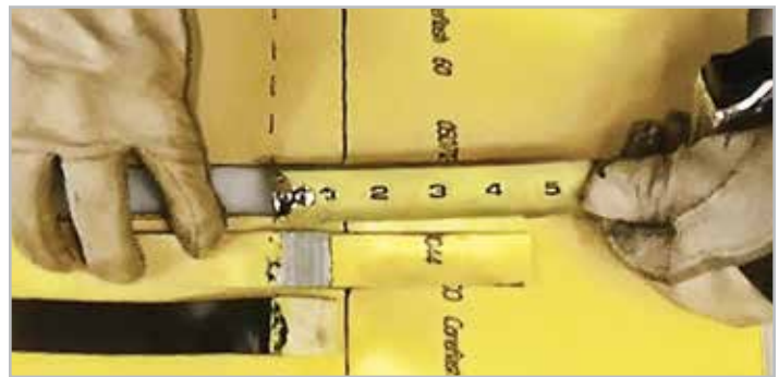
STEP 4. Weld width verification
