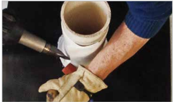
STEP 5. Weld Vertical NR to target piece
