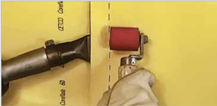
STEP 2. Pre Weld Placement
