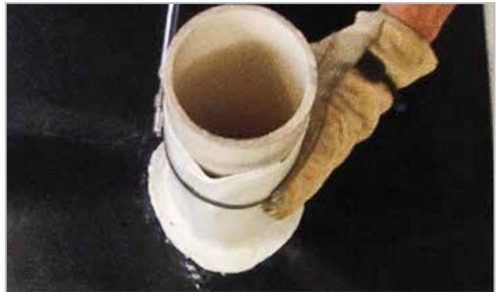
STEP 6. Install lower clamp
