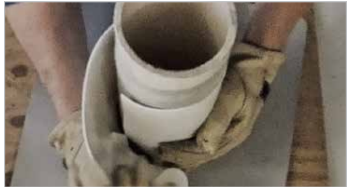
STEP 1. Place PF340 around penetration
