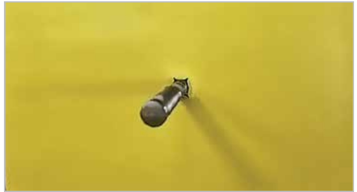
STEP 1. Install COREFLASH target piece
