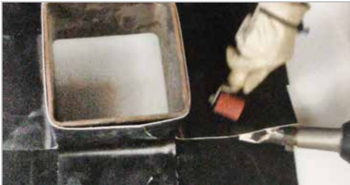
STEP 4. Weld target patch in place
