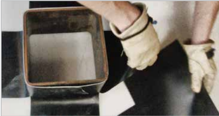
STEP 3. Place corner target patch
