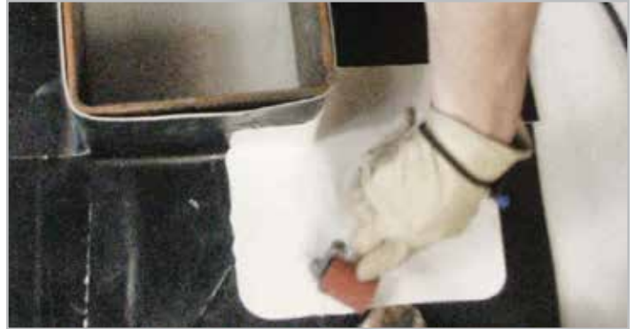
STEP 5B. Fully Weld Performed Corners to fit
