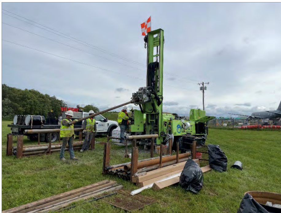
Exhibit D-3: Photo of Sonic Drill Rig at Exploration FP-MW4 (View Direction is North)
