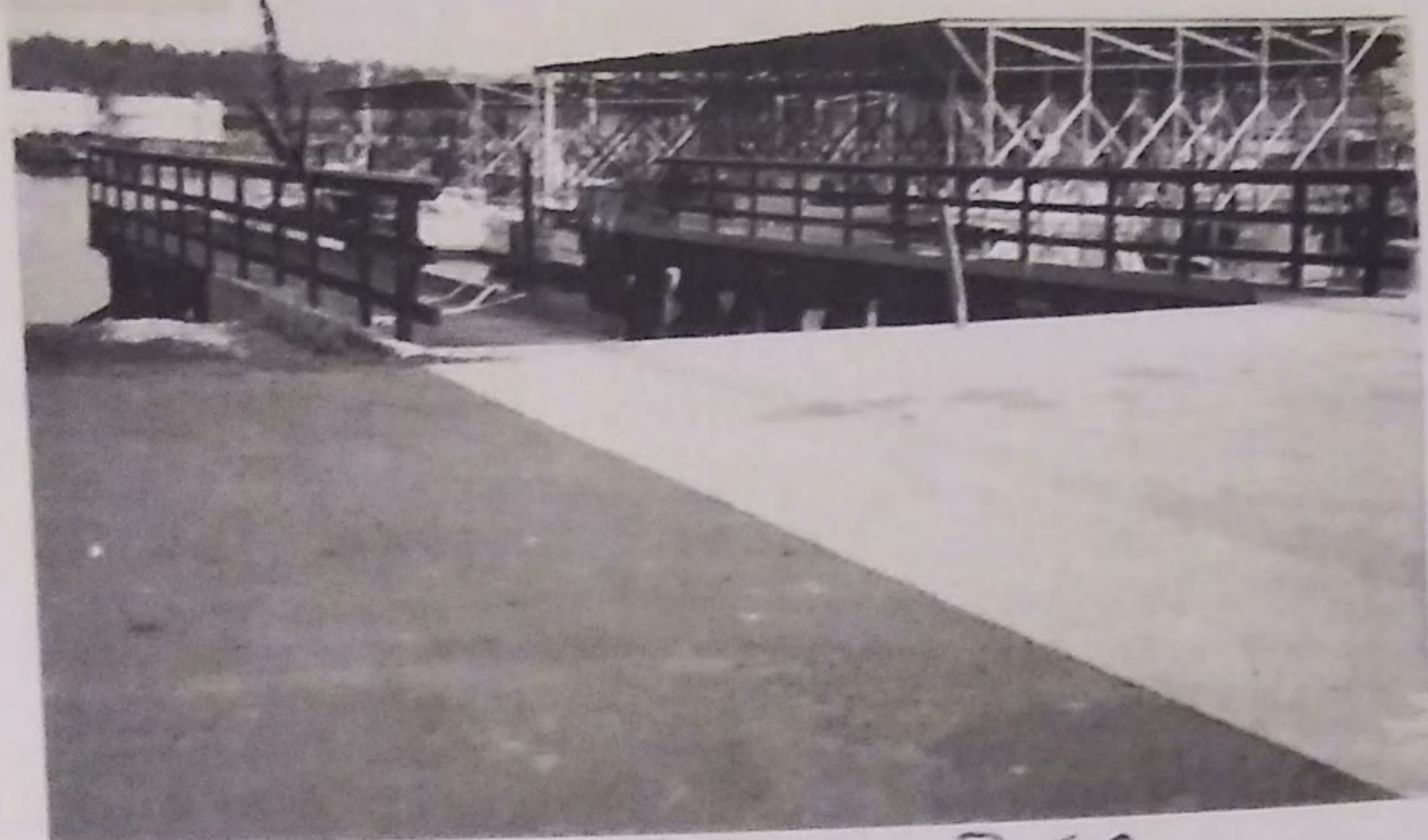
0001 TRAVELING LIFT PIER
