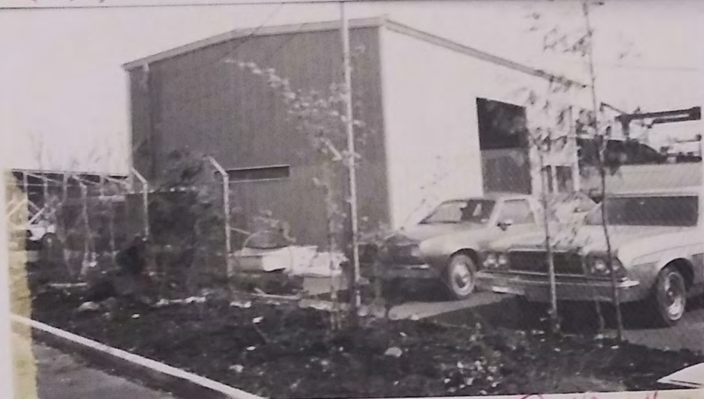
0002 STORAGE BLDG (2) 40x24
