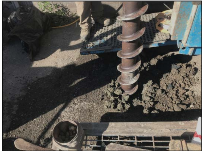
Whitty's Chevron 370 West 5 th Avenue, Colville, Washington
