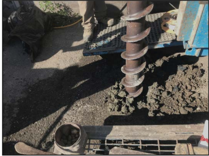
Whitty's Chevron 370 West 5 th Avenue, Colville, Washington
