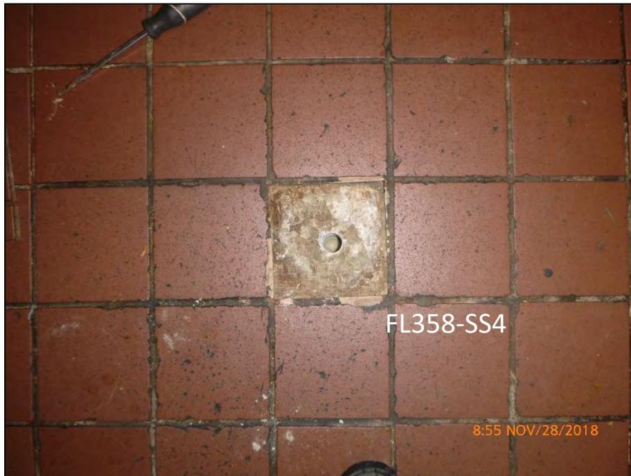
Photograph 2 – Detail of 1-inch hole advanced in slab at sample location SS4 in preparation of sampler installation.
