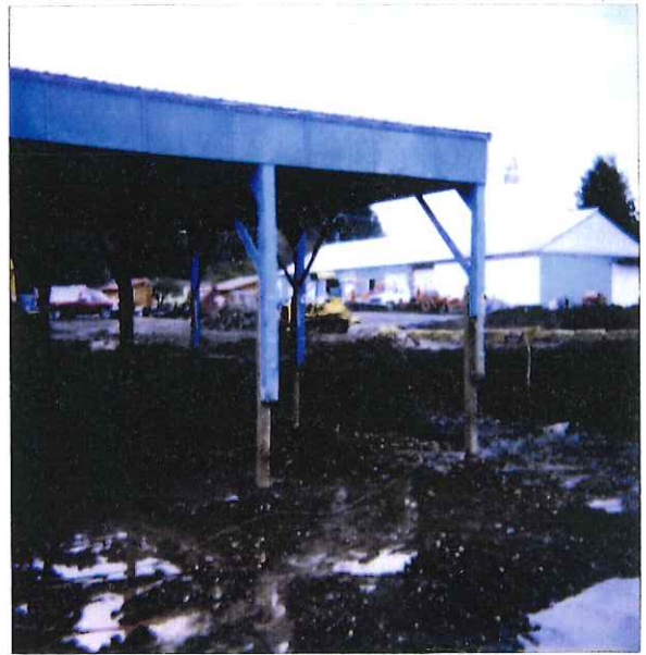
Support beams/Excavation photos
