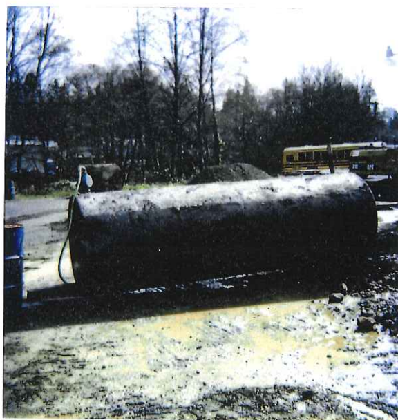
Tank #1 (gasoline leaker)
