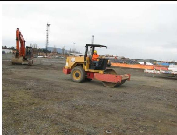
RAM Construction compacting crushed rock base course w/ 8-TON Roller.
