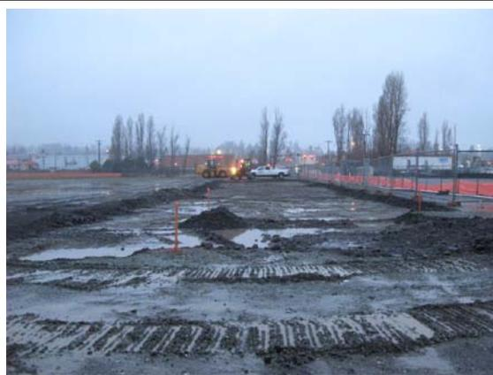
RAM Construction compacting CSBC over quarry spalls at MJB-4.
