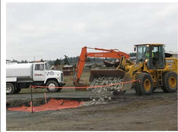
RAM Construction placing quarry spall backfill at MJB-4.
