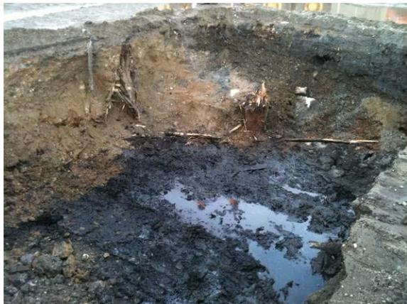
20' by 30' area RA11b excavated to 6 ft below ground surface (bgs). Looking NW. Concrete stormwater pipe in NW corner .
