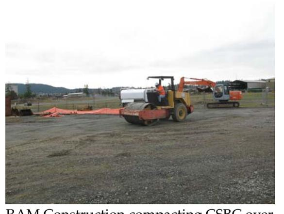
RAM Construction compacting CSBC over quarry spalls at MJB-4.
