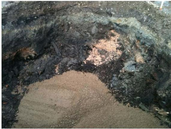
RA11a after filling up from 10 to 6 feet bgs with clean backfill pit run.
