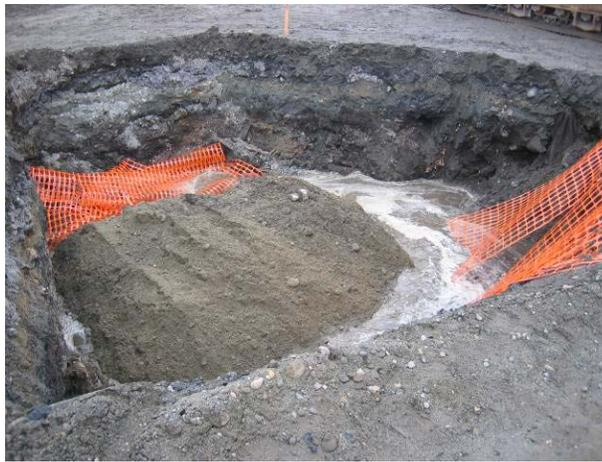
Filling in RA11a excavation with clean material on top of orange construction fence. Material was placed to existing grade and compacted.
