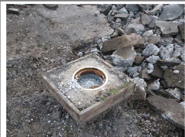
Monitoring Well ID AKL272 decommissioned with Bentonite chips. Well tag removed by driller for return to Dept of Ecology.
