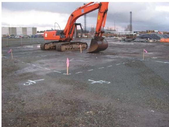
MJB-4 Excavation Re-Surveyed. 5' off-sets and excavation layout marked on ground surface.
