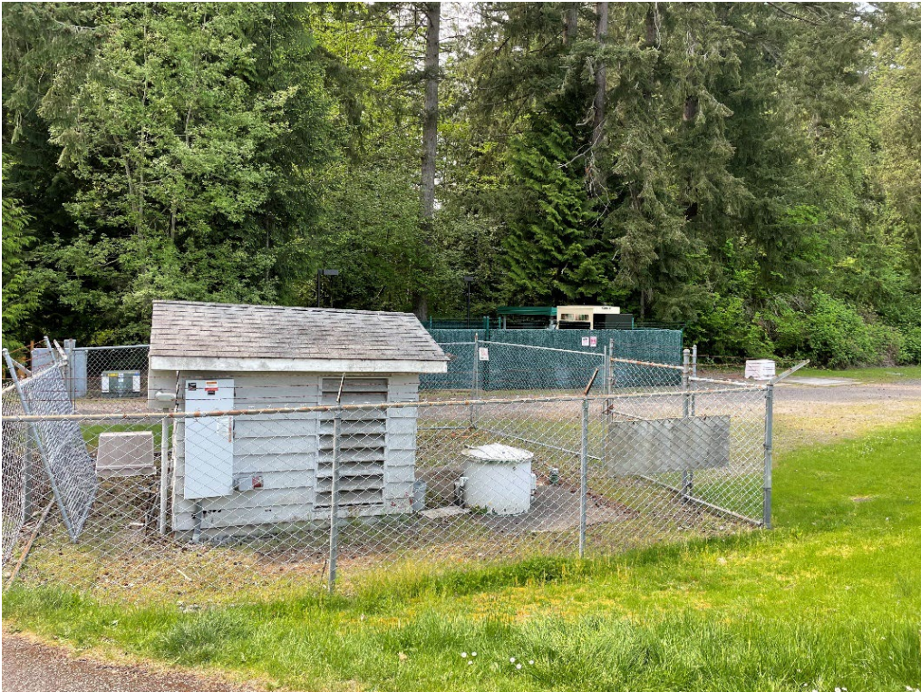
Photo 7: Lift station, facing West.
