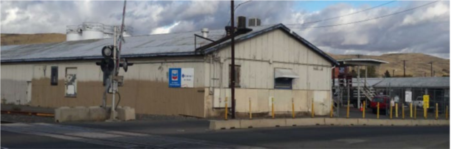
Coleman Oil Yakima Bulk Plant
