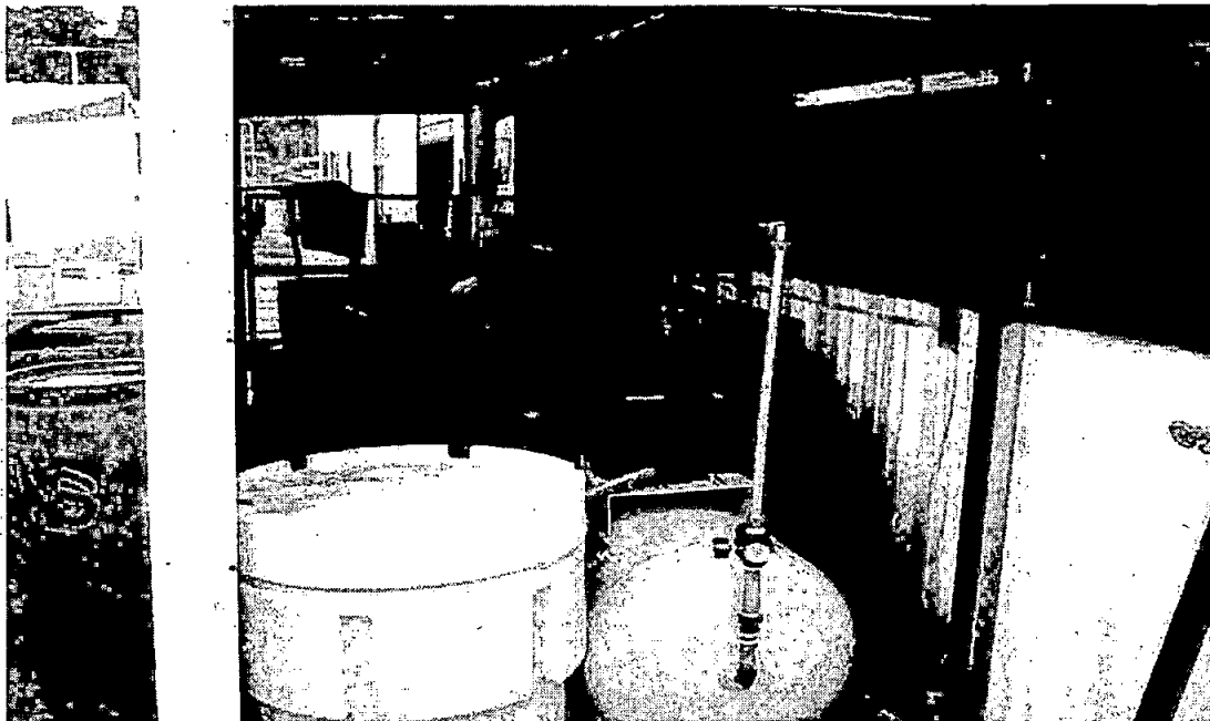
View of two ASTs (far side of shed), compressor, and white container of spill absorbent within storage shed on north side of north building. ASTs are situated within a steel containment. Blue drum at left of photo was empty.
