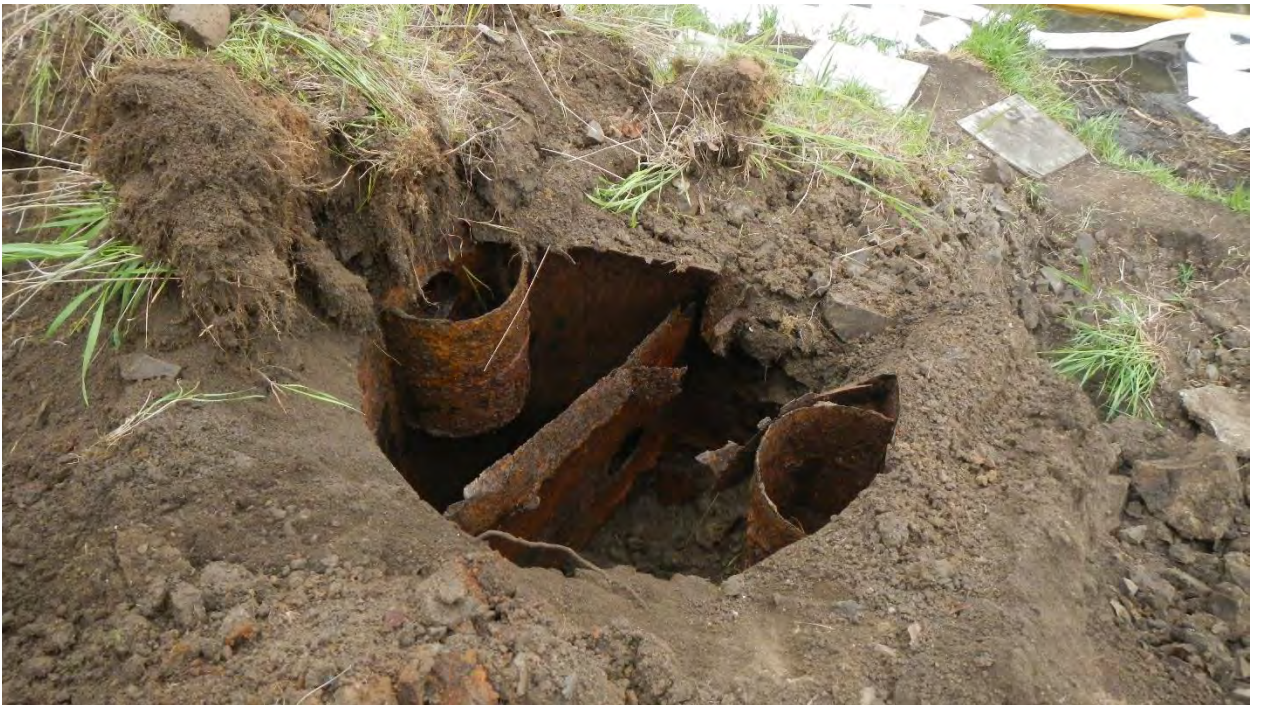
Figure 9. Overview of the oil/ water separator. View to the north.
