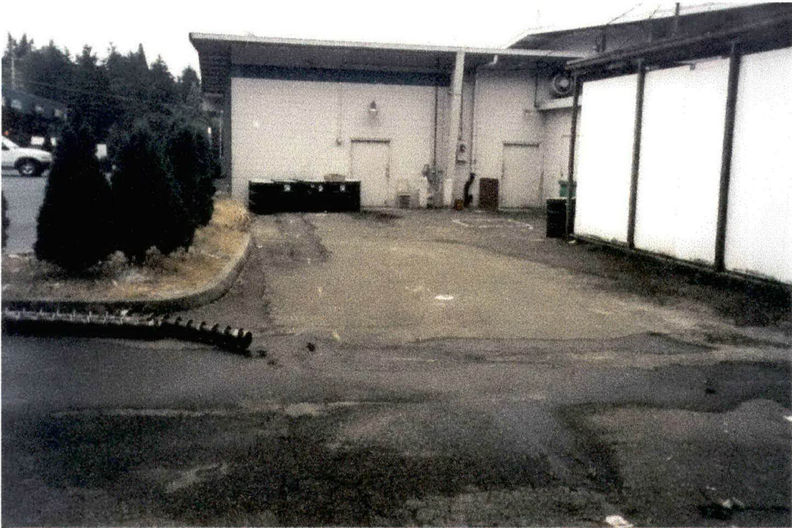
Photo 7. View to the east showing the rear entrance to the dry cleaner tenant space. The white painted rectangle immediately adjacent to the building marks the location of the inactive dry well that was reported to formerly drain storm water off the building roof.
