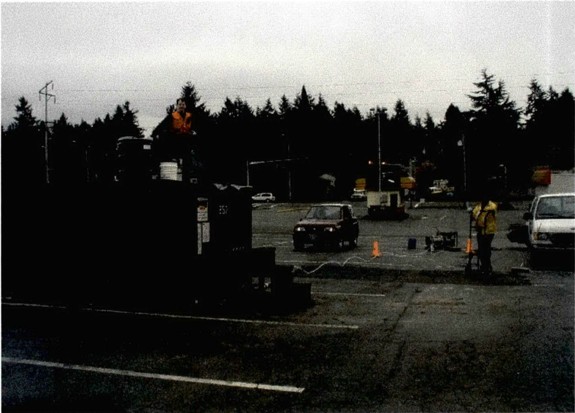
Photo 7. View towards the east during the pumping and carbon treatment of PCE contaminated water from the three 1,000 gallon septic tanks formerly located in the main parking area. The treated water was hauled to METRO water treatment plant.
