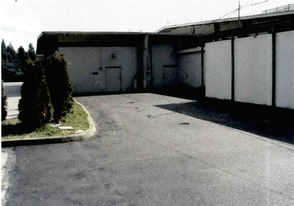
Photo 10. View towards southeast of showing the rear of the former Sooper Cleaners after completion of the remedial activities.
