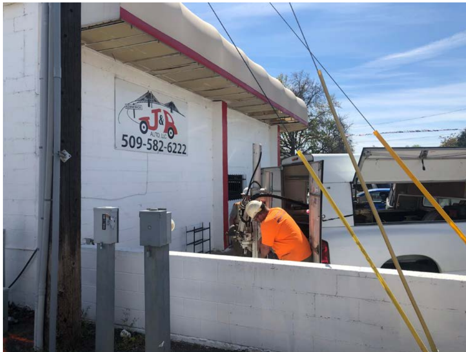
Advancing boring location GEI010-DP4 (view looking south)
