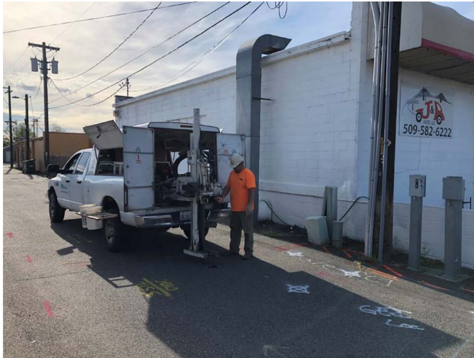
Advancing boring location GEI010-DP1 (view looking east).
