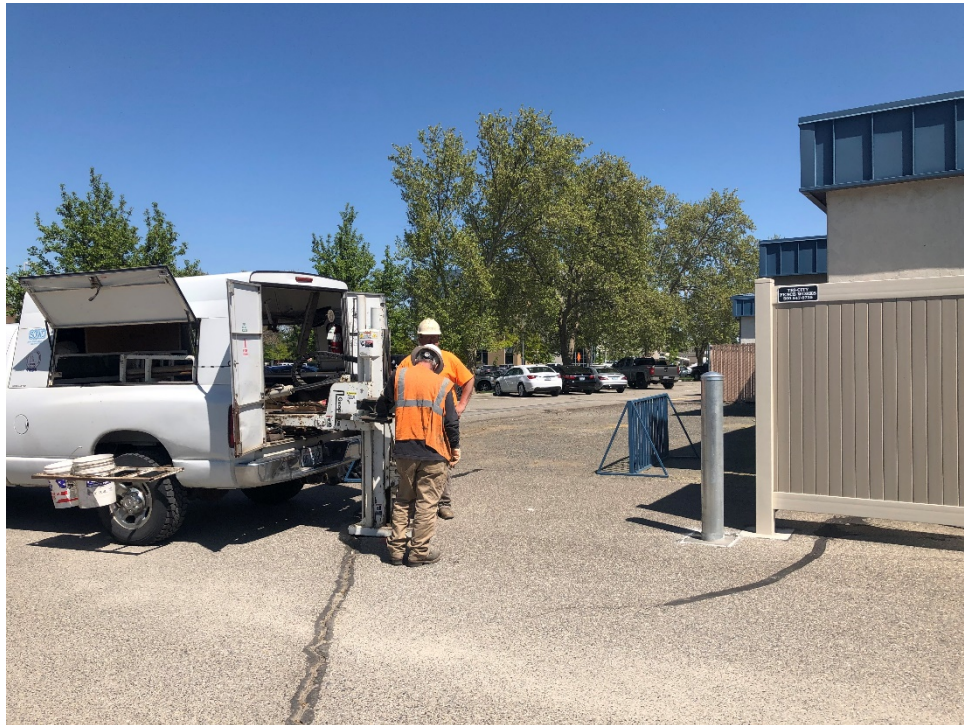
Environmental West advances soil boring GEI009-DP1 (view looking east).
