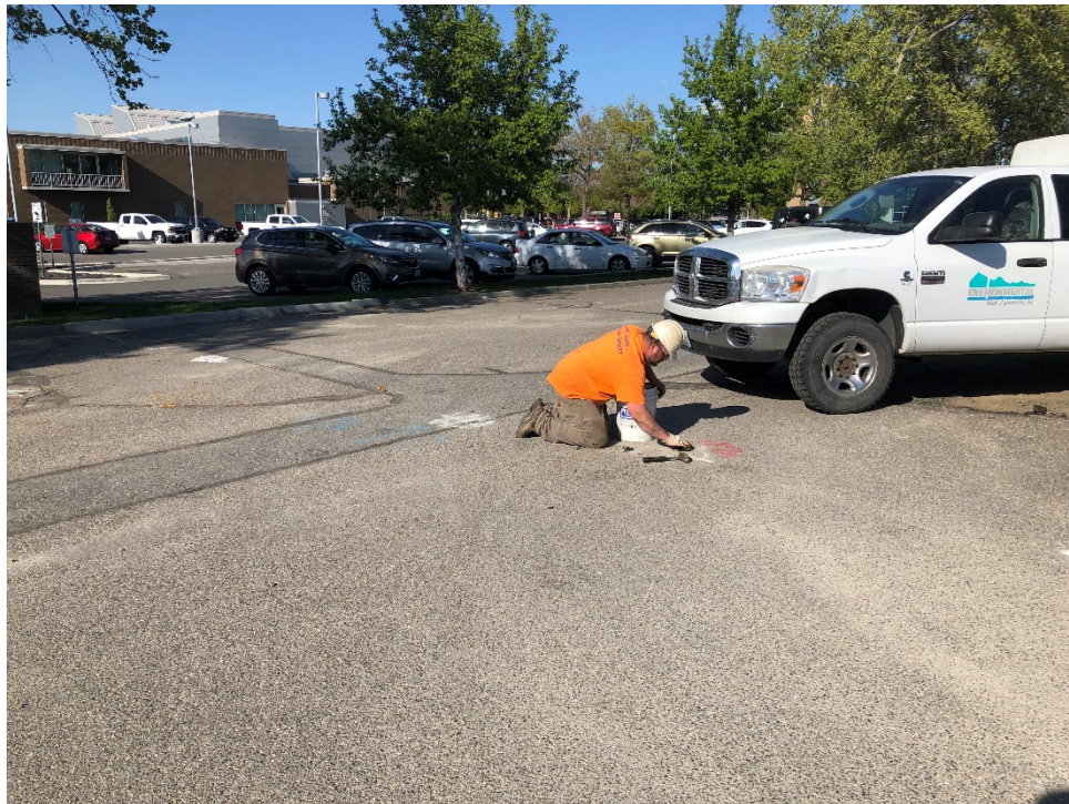
Environmental West completes GEI009-DP-5 with asphalt patch (view looking northeast)
