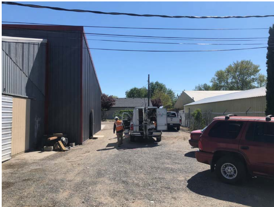
Advancing boring location GEI014-DP3 (view looking east)
