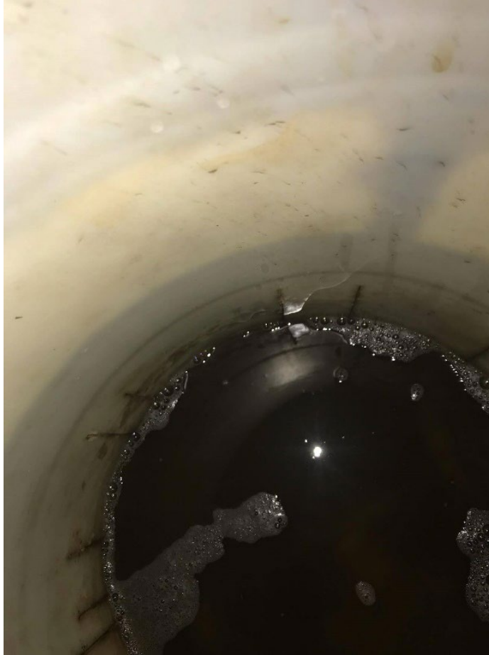
Figure 5. Interior View of Unknown Well
