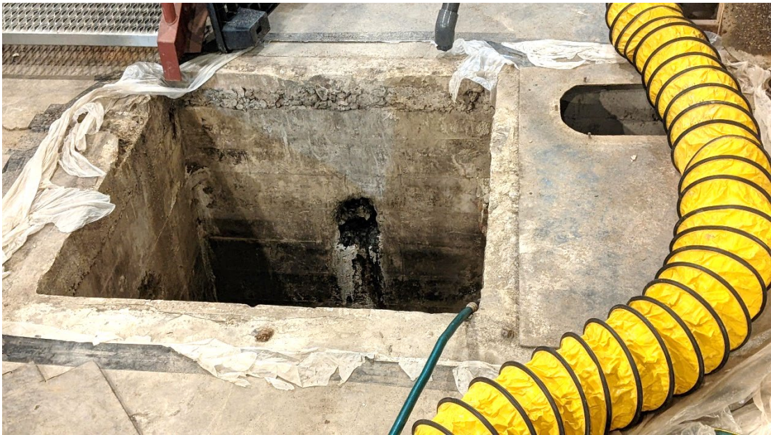
Figure 9. Surface Access to Main Sump and Small Sump
