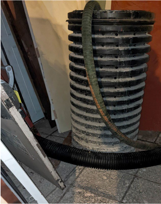
Figure 6. Exterior View of Drywell
