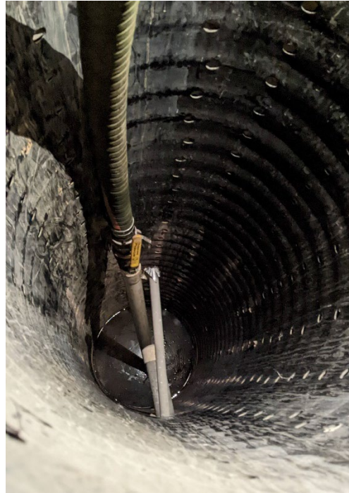
Figure 7. Interior view of Drywell
