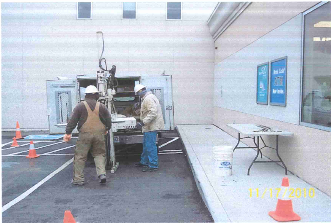
PUSH-PROBE SAMPLING AT THE FORMER HOT LOCATION .
