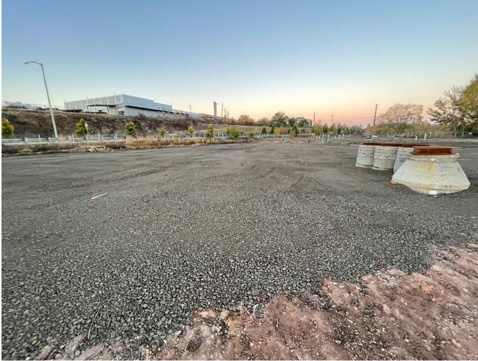
Photograph 3. View of proposed Building 2B footprint with building footprint excavation backfilled and stormwater cover placed and compacted. Looking west.
