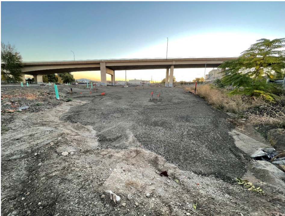
Photograph 4. View of proposed Building 2B footprint with building footprint excavation backfilled and stormwater cover placed and compacted. Looking east.
