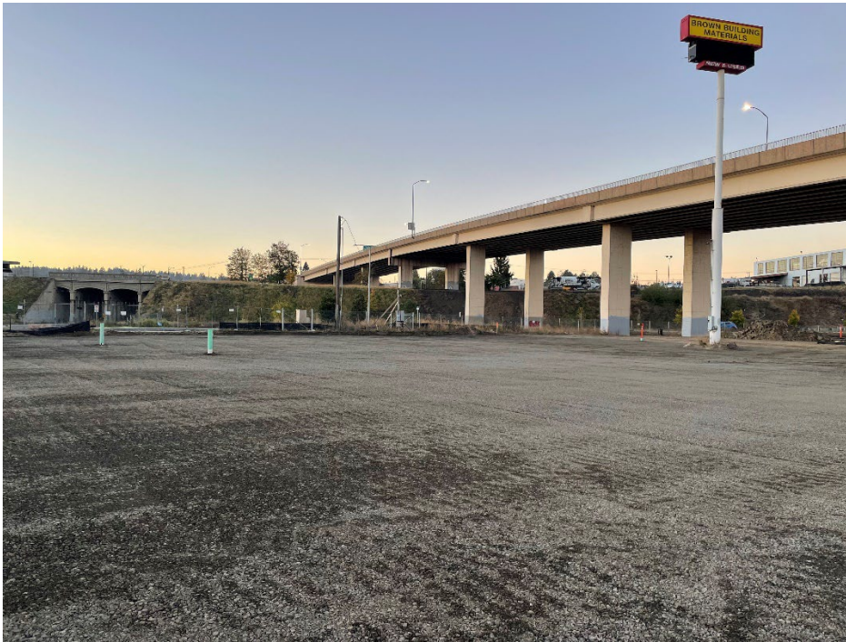
Photograph 2. View of proposed Building 2A footprint with building footprint excavation backfilled and stormwater cover placed and compacted. Looking southwest.
