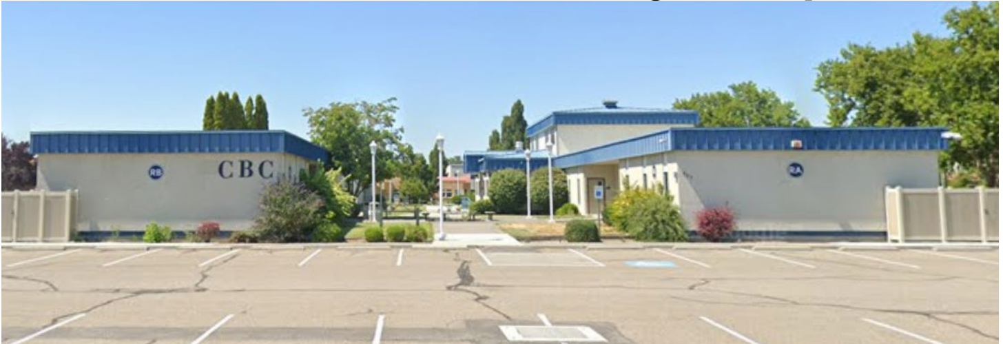
CBC WSU Nurse Training Facility – Photo courtesy of Google Street View
