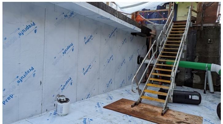
SV.04.02.B - View of horizontal to vertical transition of membrane
