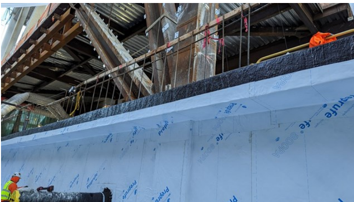
SV.04.02.C - Top of east wall termination
