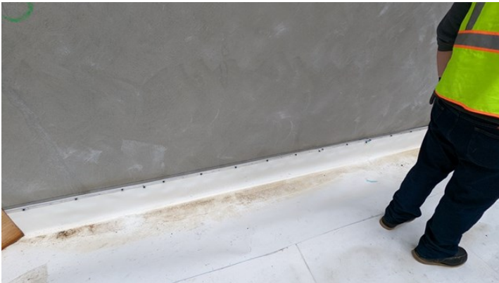
SV.02.02.A - Typical perimeter termination with term. bar
