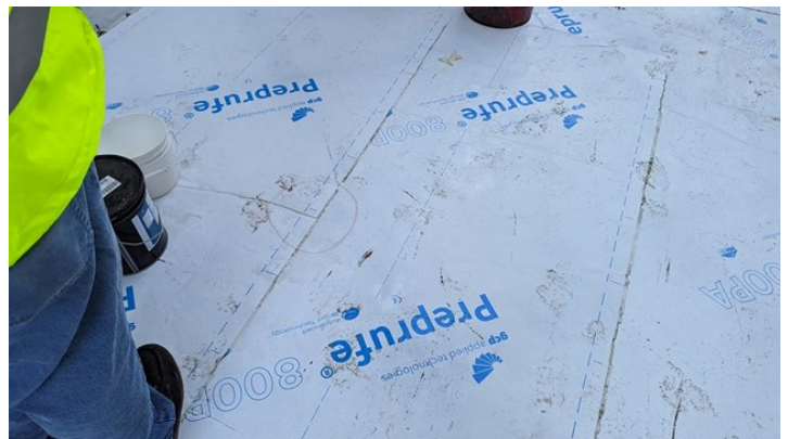
SV.04.02.D - Fishmouth marked for repair by Sound waterproofing
