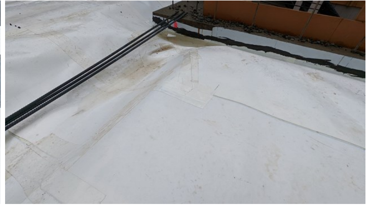
SV.02.01.F - Additional tape applied at location indicated by GCP
