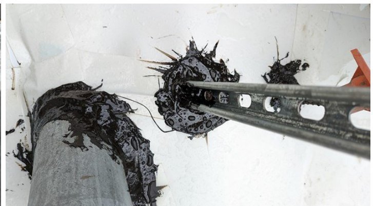
SV.02.03.D - Overview of pipe penetration
