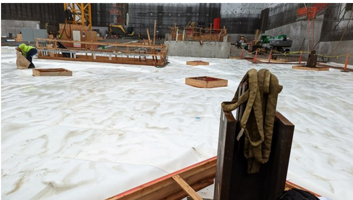
SV.02.01.C - Overview of vapor barrier installation
