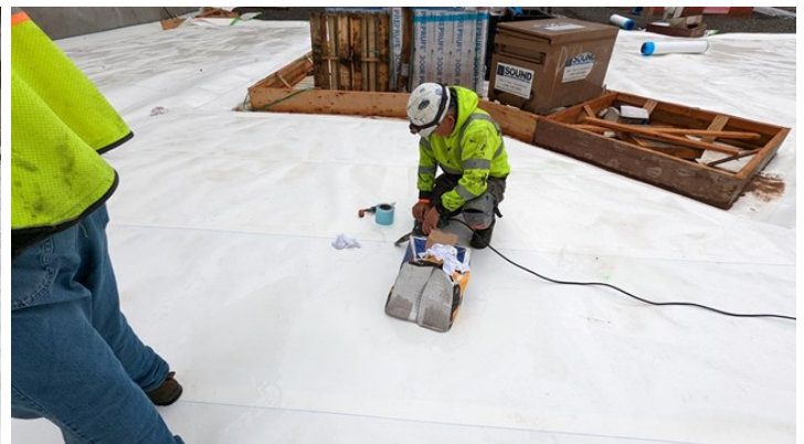
SV.02.01.D - In progress vapor barrier sealing
