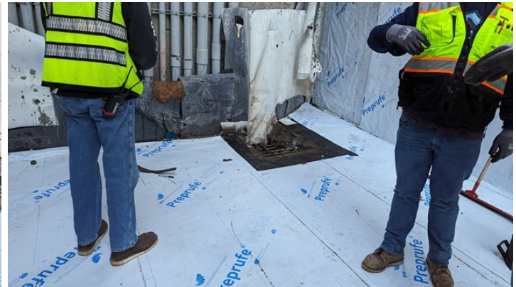
SV.04.05.B - Overview of leave out in slab
