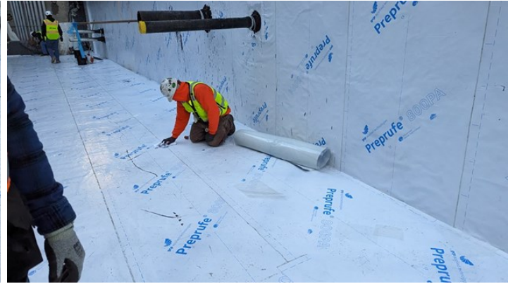
SV.04.02.F - View of membrane cleaning prior to installation of membrane patch
