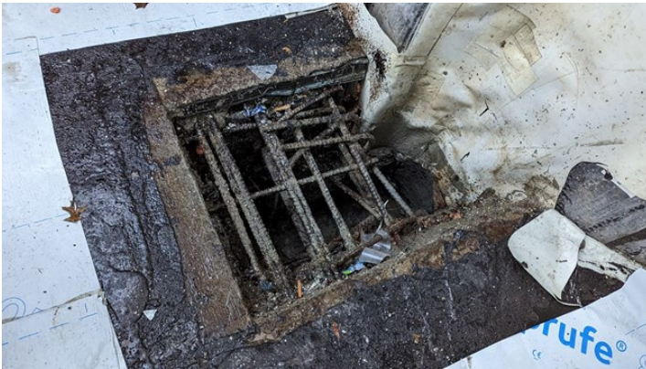
SV.04.05.A - Overview of leave out in slab
