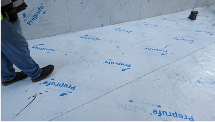
SV.04.02.E - View of patch repair
