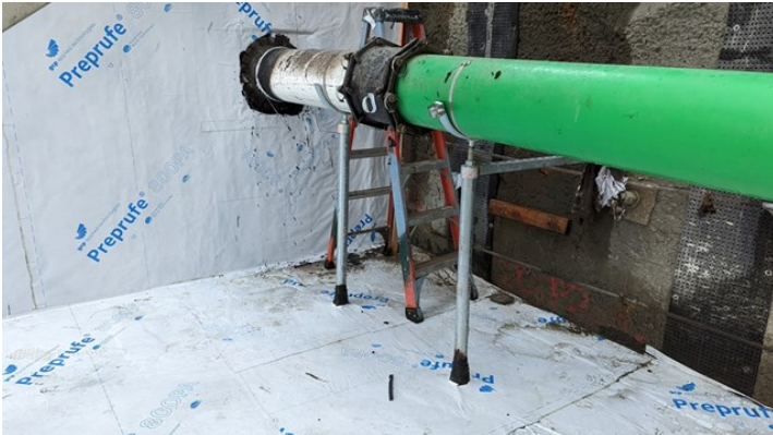
SV.04.03.A - Example of typical pipe penetration detailing
