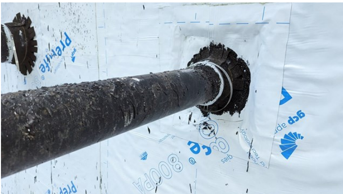
SV.04.03.C - Example of typical pipe penetration detailing
