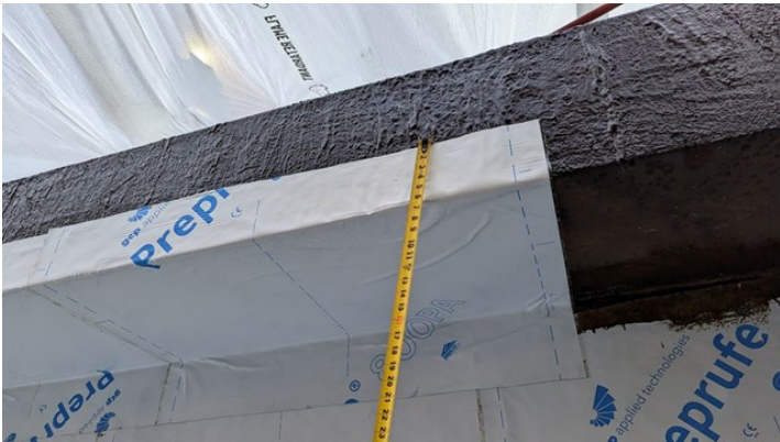
SV.04.04.E - Extent of preprufe installation onto vertical wall above.
