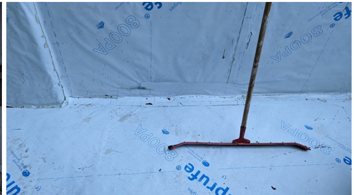
SV.04.04.B - Typical vertical to horizontal transition
