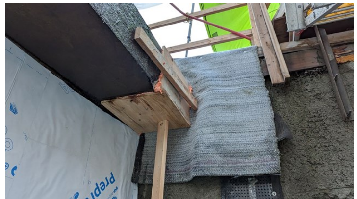
SV.04.04.H - Transition at south side of area reviewed
