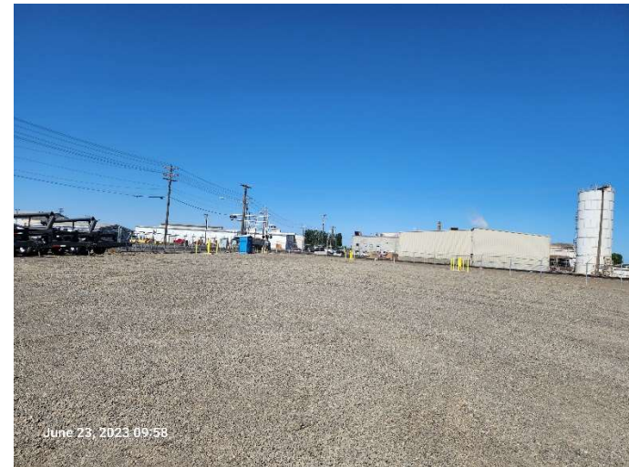
Photo 36. Looking west at all completed new wells
