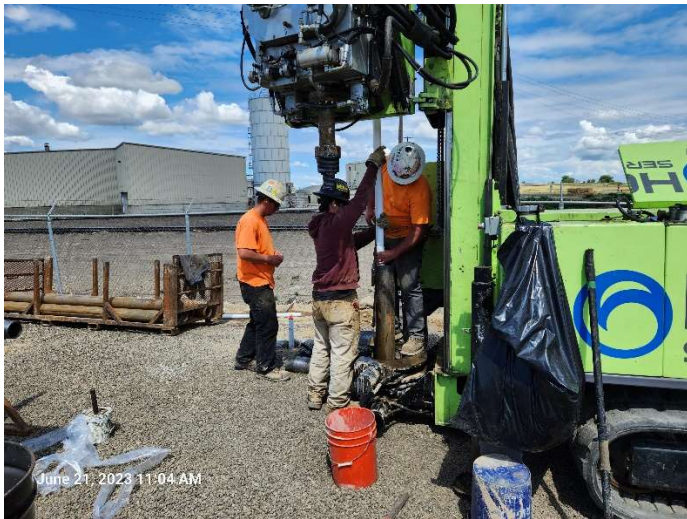
Photo 25. PVC placement at MW-5SR
