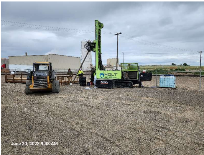
Photo 27. Drilling at MW-5DR
