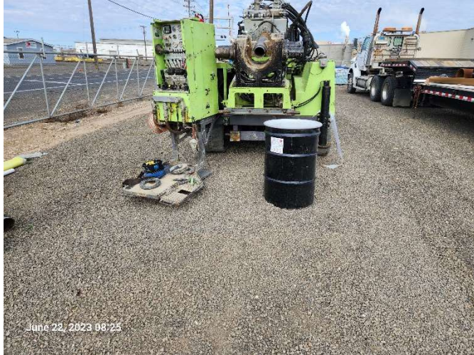
Photo 1. Drill rig setup/location at MW-11S
