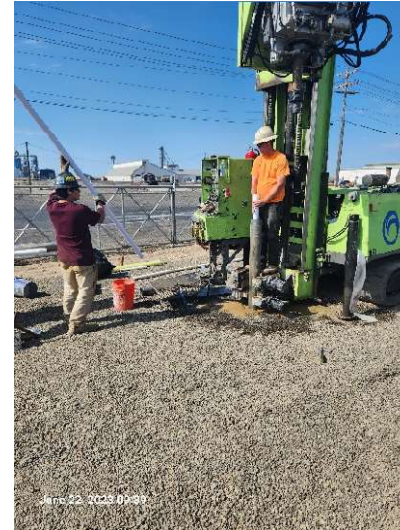
Photo 10. MW-11S PVC placement
