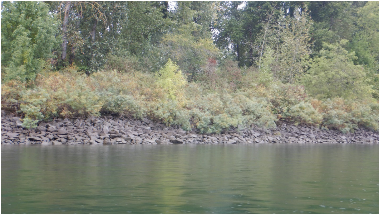
Photograph 2-2 Shoreline Segment Along Southeast Lady Island: Engineered Riprap
