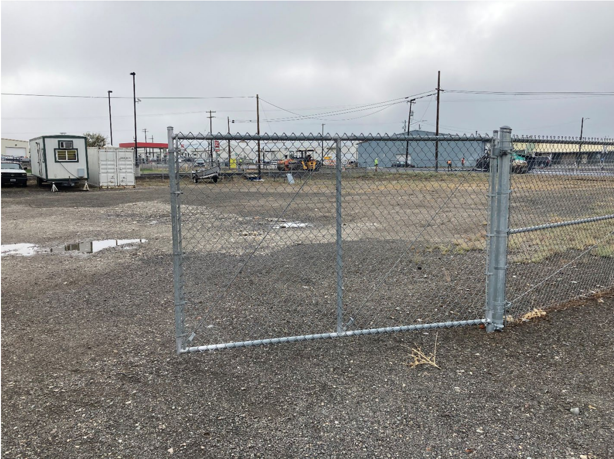
Photo 6: Gate to the City Parcel property (open for site inspection)
