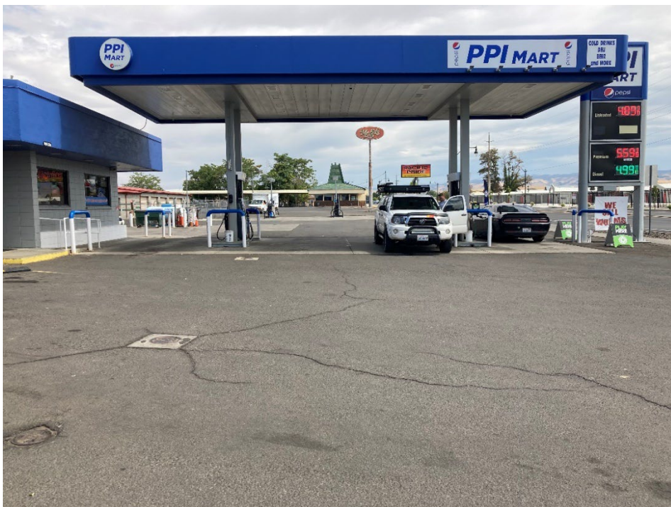
Photo 2: Fuel pump canopy—from the west
