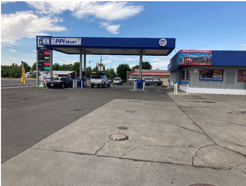
Photo 4: Fuel pump canopy and convenience store—from the east
