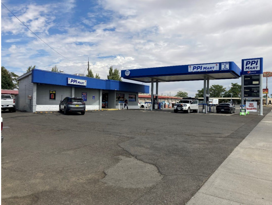
Photo 1: Street view of Site—from the south
