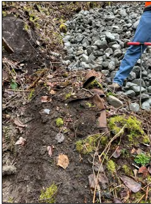
Photograph 11. Additional view of metal debris discovered upslope of weir box.
