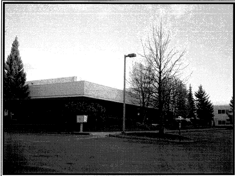
Figure 17 Rental No. 3 Green River Corporate Park Building A 20416 72 nd Avenue South
