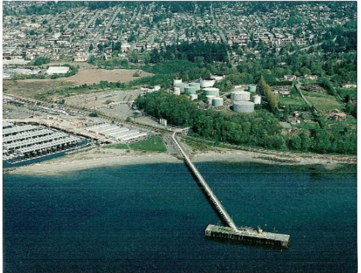
Historic view of fuel terminal
