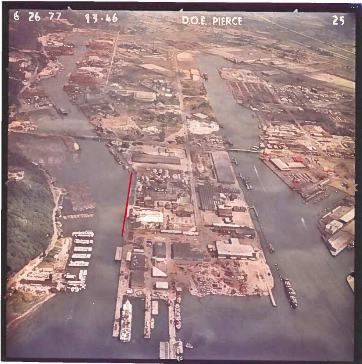
Figure 17. 1977 aerial imagery of the Blair-Hylebos peninsula annotated with the location of the proposed barrier wall (red line) (WAECY 2020c).
