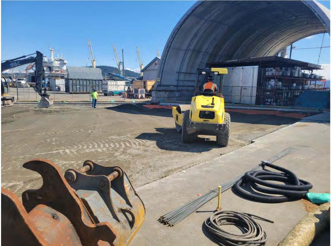
Image 1 - Compaction of CSTC
