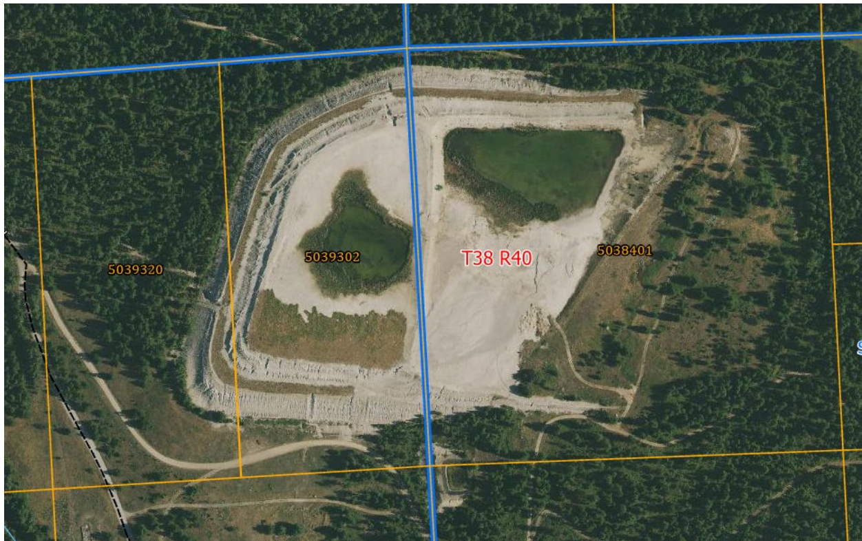
Figure 1. Lower Tailings Pile with corresponding parcel numbers.
