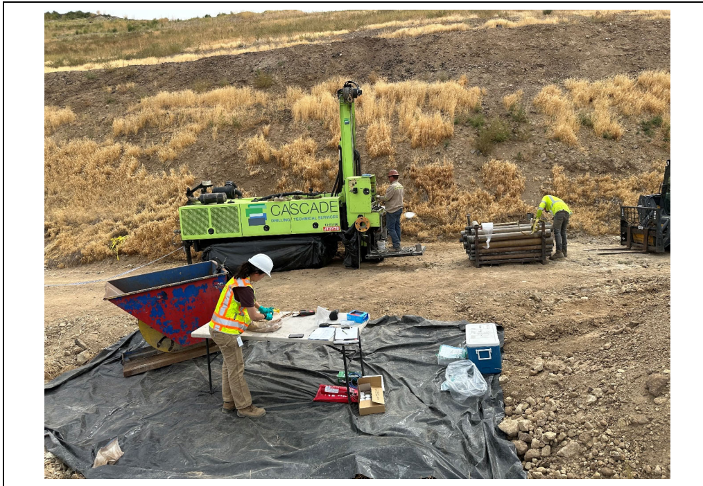
Cascade conducting sonic drilling and Parametrix field personnel observing soil samples.
