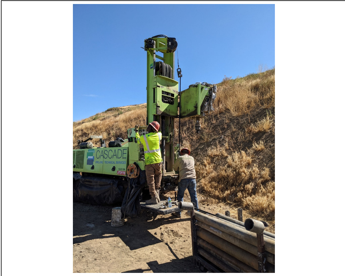
Installation of thermistor and gas probe at site T2.
