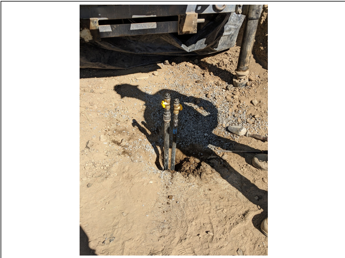
Completed installation of thermistor and gas probe at site T3.
