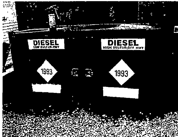
Photo 11 – Cabinet containing diesel fuel with soil staining.
