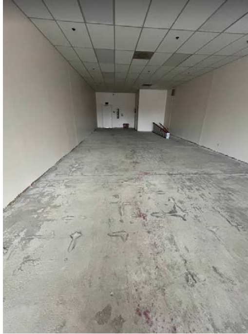
Photograph 15. Floor Slab and Ceiling in Suite B7 (December 8, 2023)
