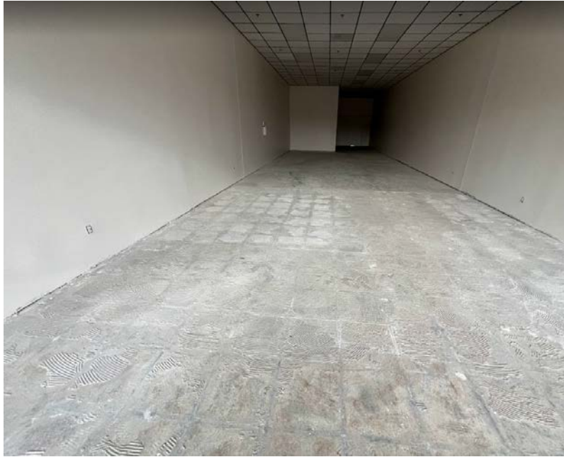
Photograph 1. Floor Slab in Former Harbour Pointe Cleaners (Suite B6) (December 8, 2023)
