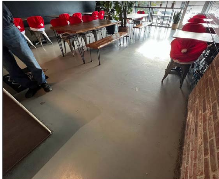
Photograph 8. Floor Slab in Adjacent-West Tenant Space (Suite B5) (December 8, 2023)
