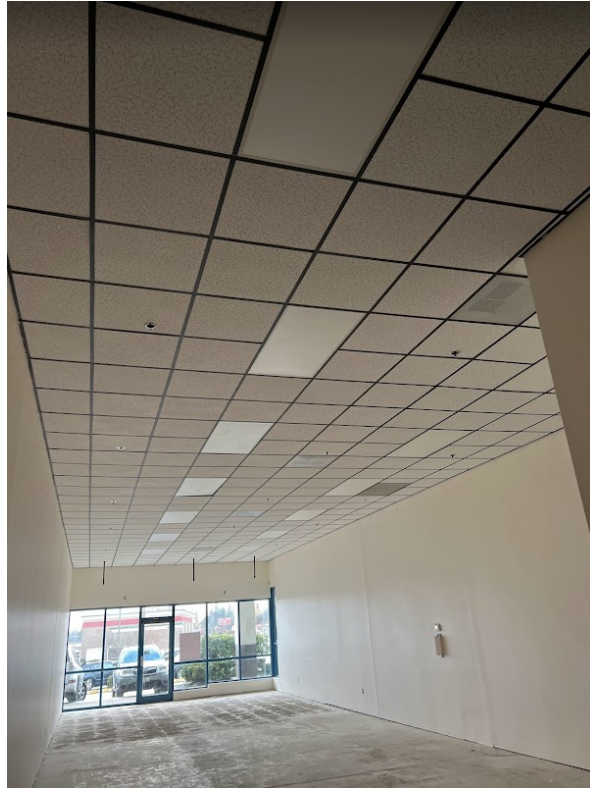
Photograph 7. Ceiling of Former Harbour Pointe Cleaners (Suite B6) (December 8, 2023)
