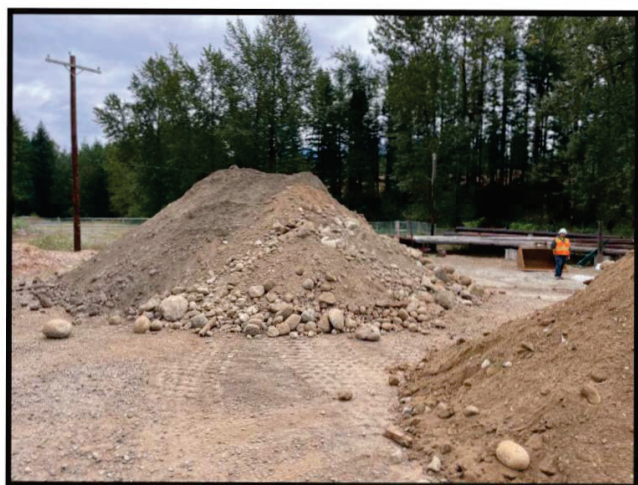
Imported clean fill and excavated fill material (excavated soil contains TPH detections up to 250 ppm)
