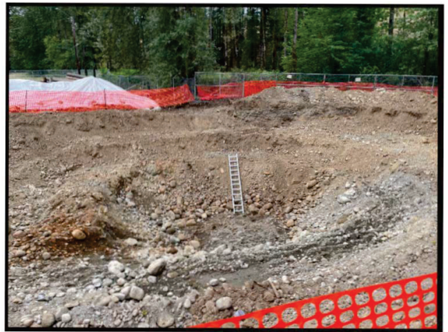
Excavation pit ~20 ft deep still encountering >5000 ppm
