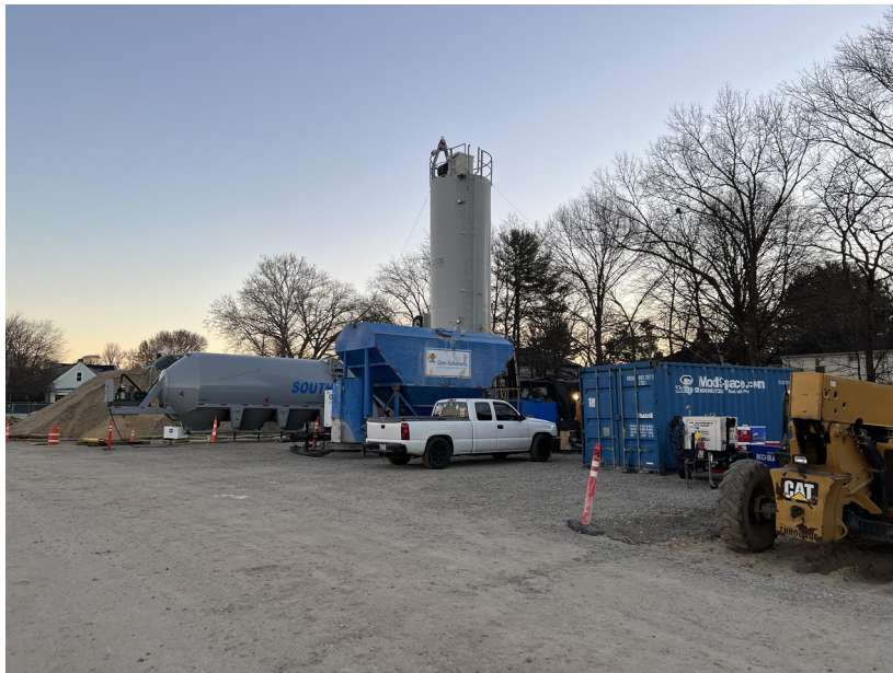
Photo 6-2: ISS batch plant.
