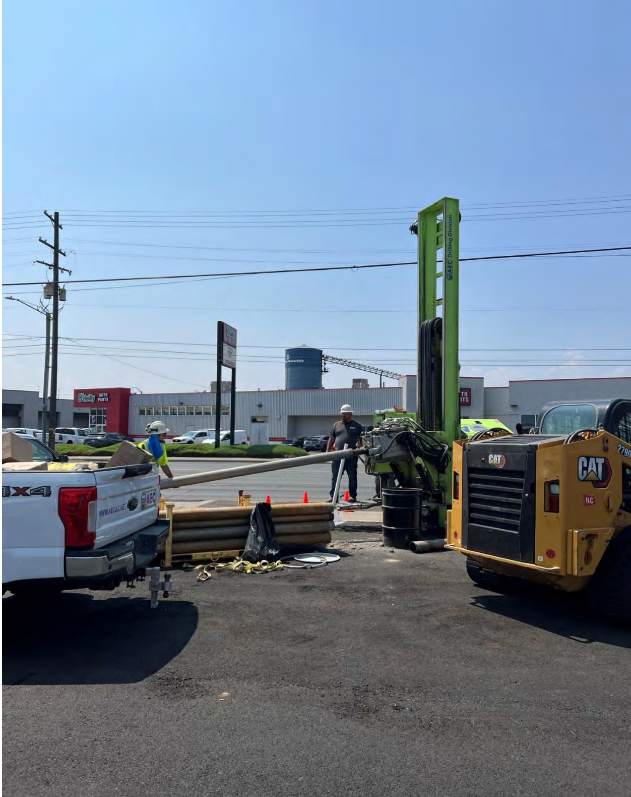
Photograph 5 – Terra sonic drilling rig set-up to advance boring MW9 on May 19, 2023 (facing west).
