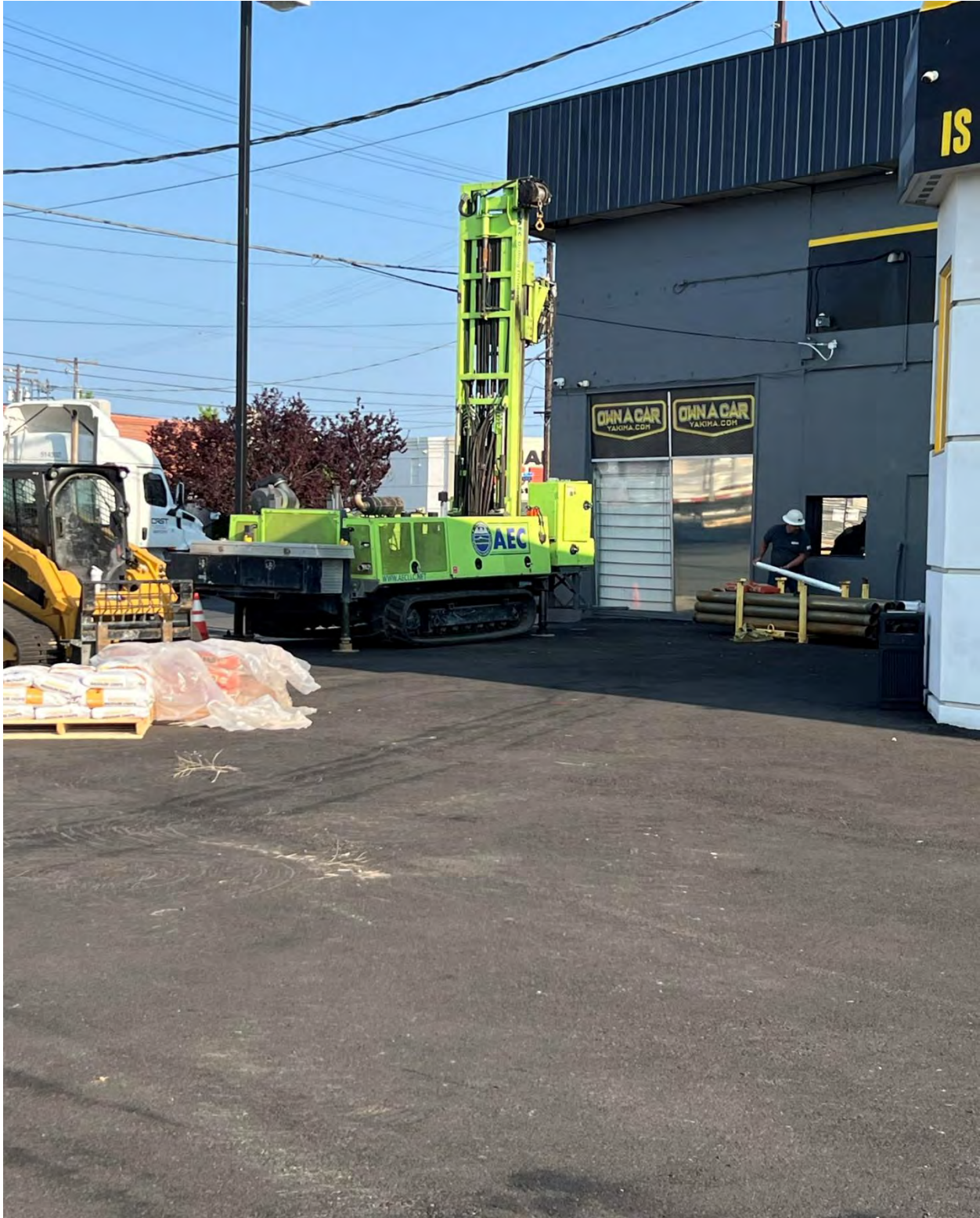
Photograph 1 – Terra sonic drilling rig set-up to advance boring MW7 on May 19, 2023 (facing NW).
