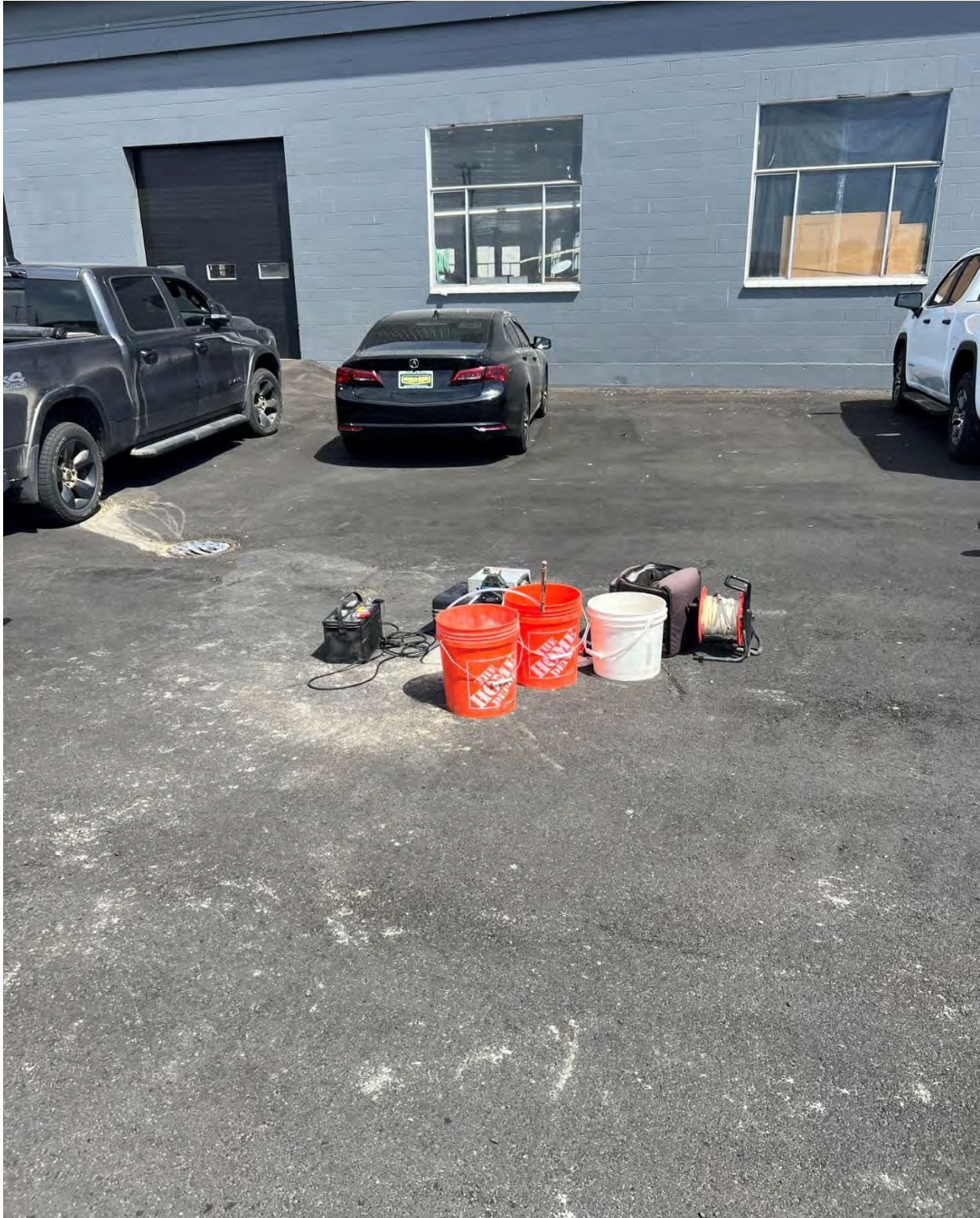
Photograph 12 – Purging groundwater from replacement well MW3A, prior to sample collection on June 13, 2023 (facing north).
