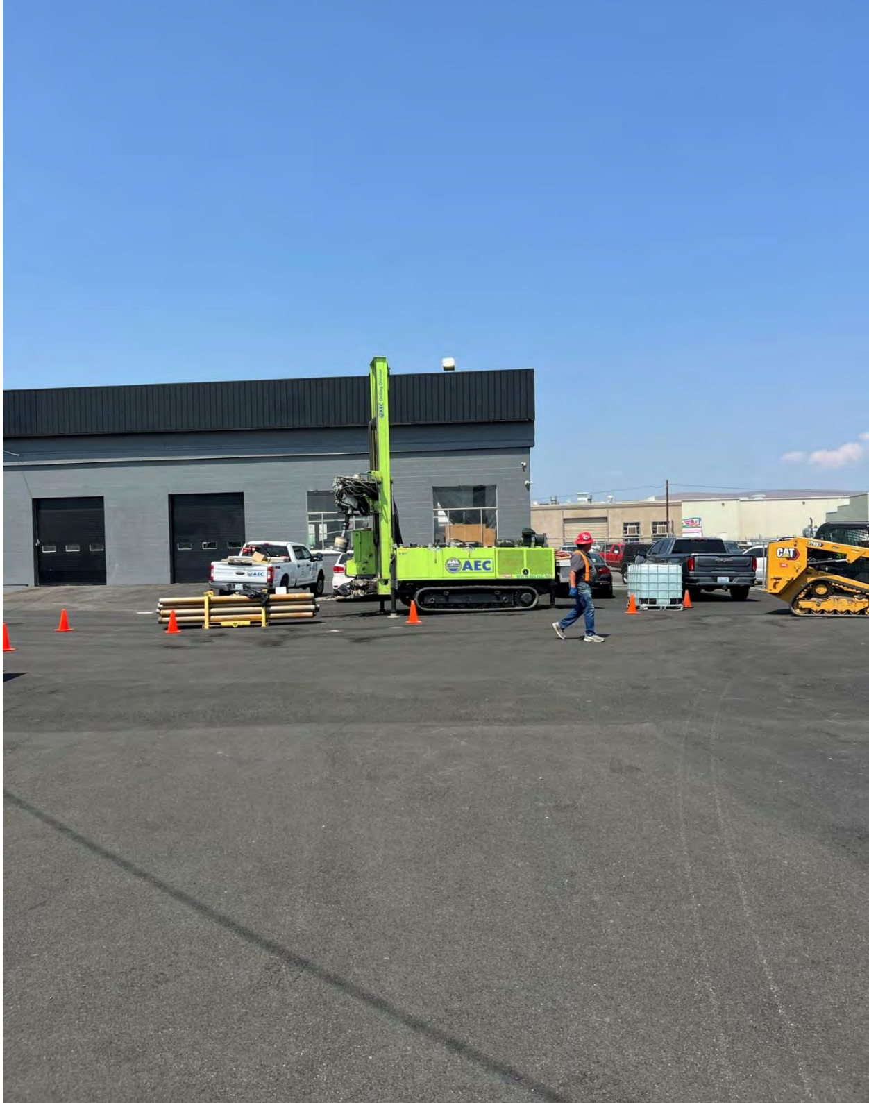
Photograph 6 – Terra sonic drilling rig set-up to advance boring MW3A on May 19, 2023 (facing north).
