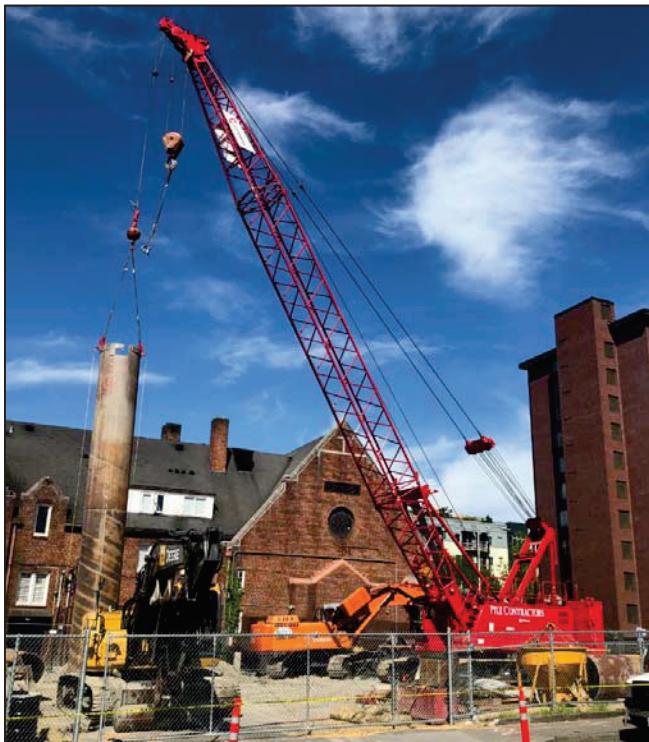
Image 6-1 Shoring Installation
