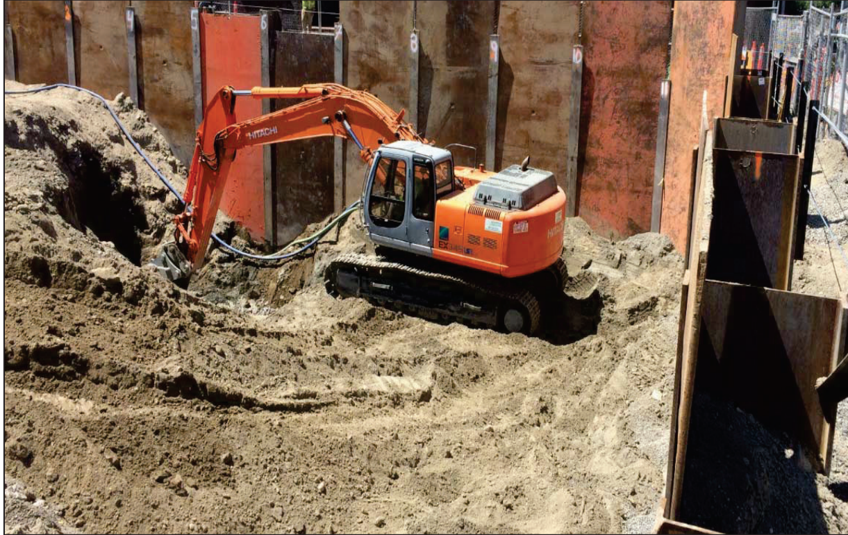
Image 8-1 Remedial Over-Excavation
