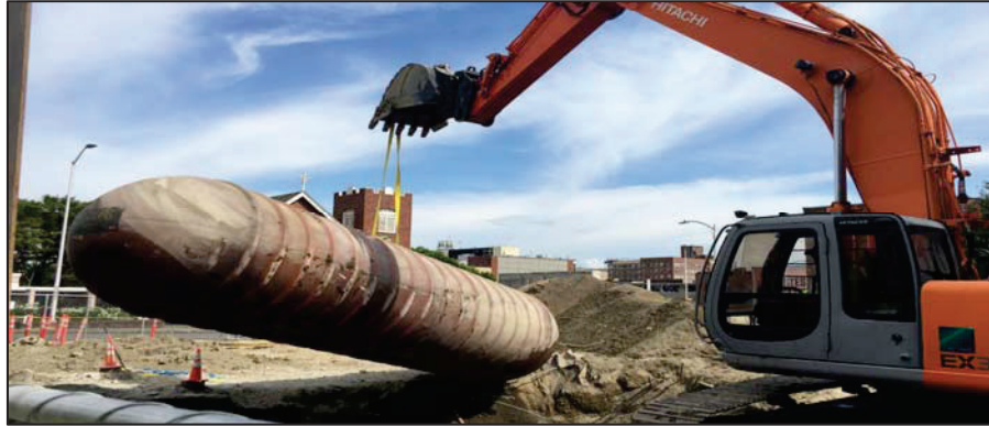
Image 7-1 Removal of Three 10,000-Gallon USTs
