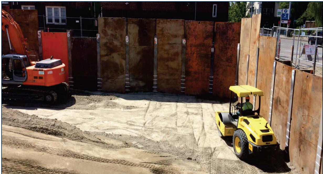
Image 8-3 Excavation Backfill and Compaction
