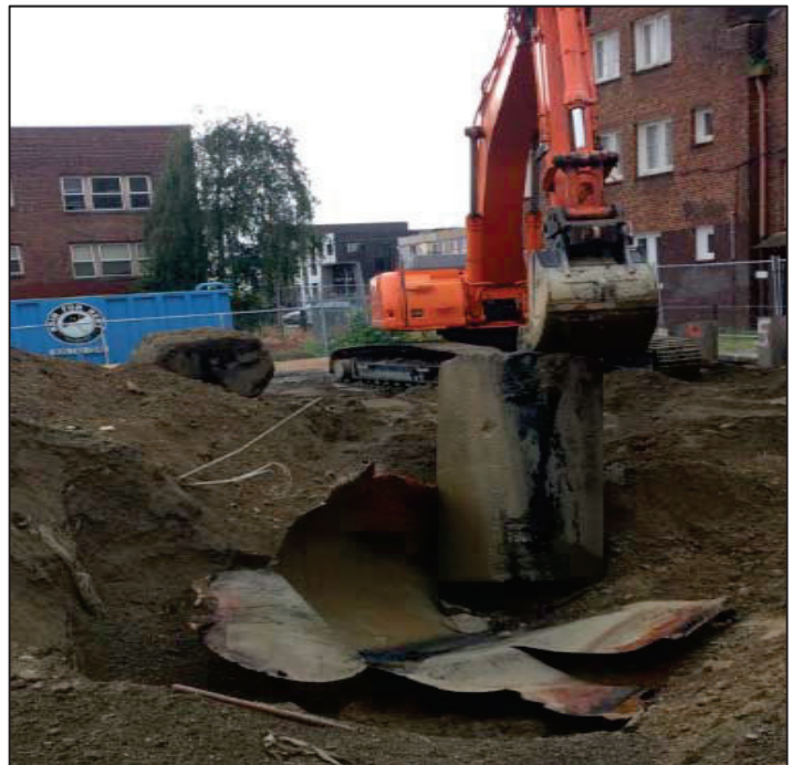
Image 7-2 Removal of Three 2,000-Gallon USTs
