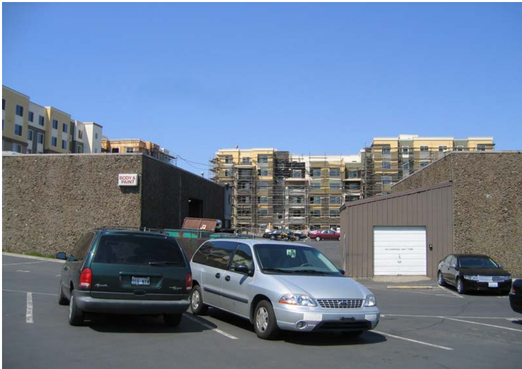
South to north view of Olympic Lincoln Mercury auto service shops in the foreground and northeast portion of the Site (building under construction in background).
