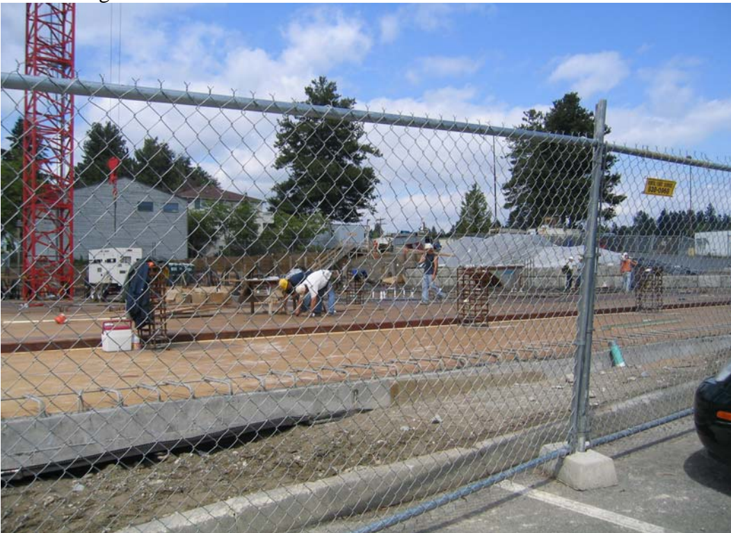
Southwest to northeast view of the Site.
