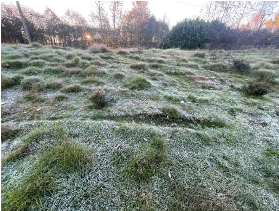
Photograph L7. Stations LLA 15 during the November 16, 2023, follow-up barrier inspection. Improved conditions due to increased vegetation were noted; barrier repair is not required. See Photograph L6 for previous conditions.
