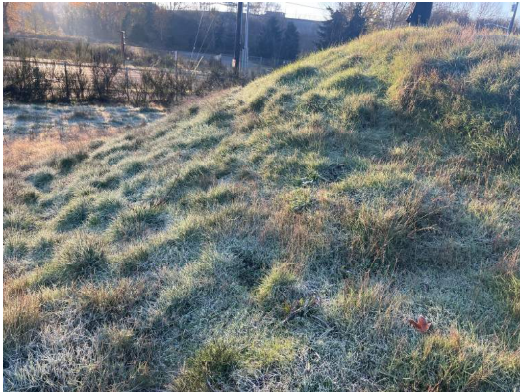
Photograph L2. Station LLA 02 during the November 16, 2023, follow-up site inspection. Improved conditions due to increased vegetation were noted; barrier repair is not required.
