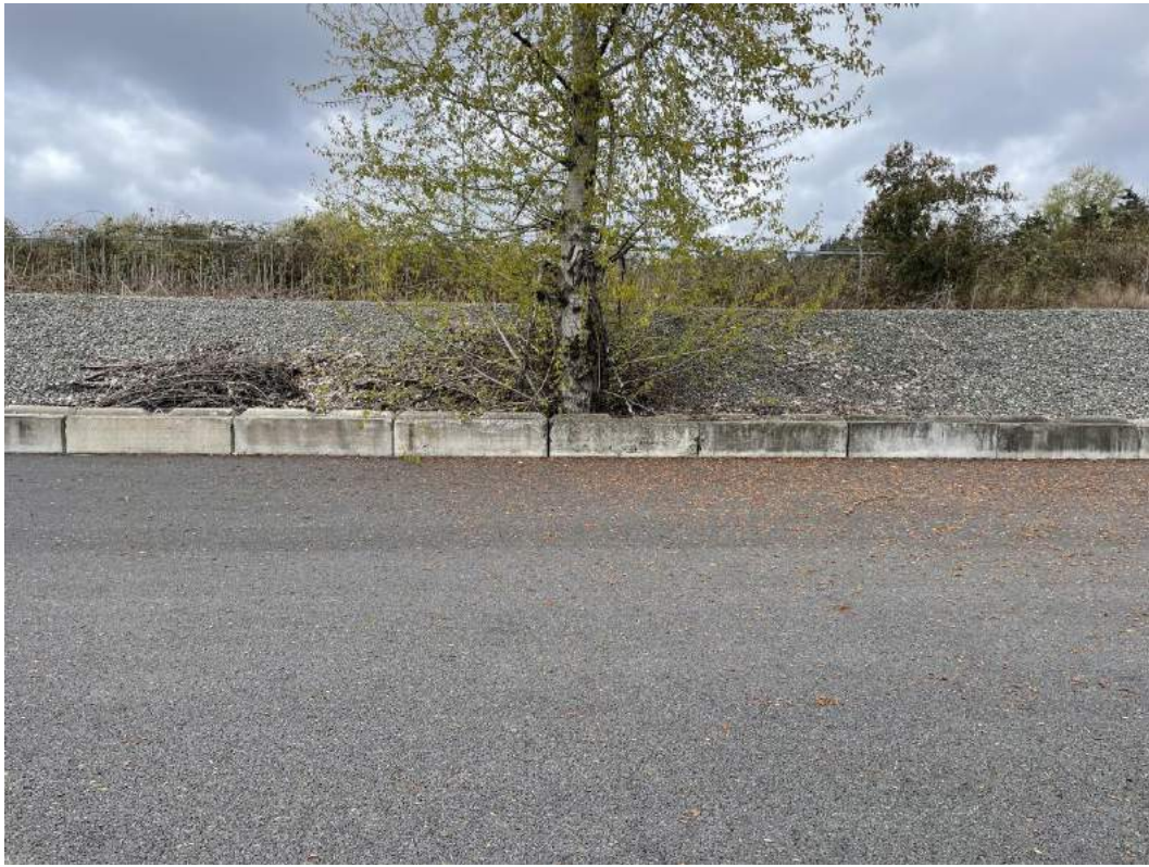
Photograph D1. Station DMCA 01 at the west border of the DMCA with organic debris and blackberry growth.
