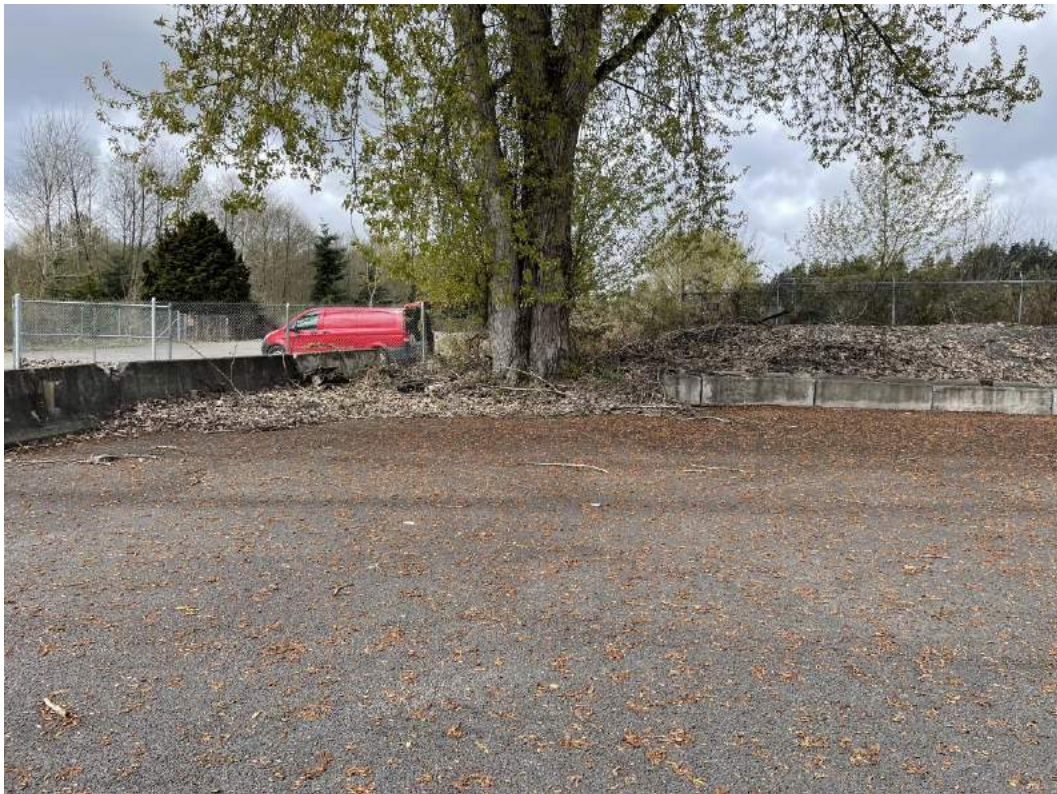
Photograph D4. Substantial organic debris at the southwest corner of the cap near Station DMCA 09.
