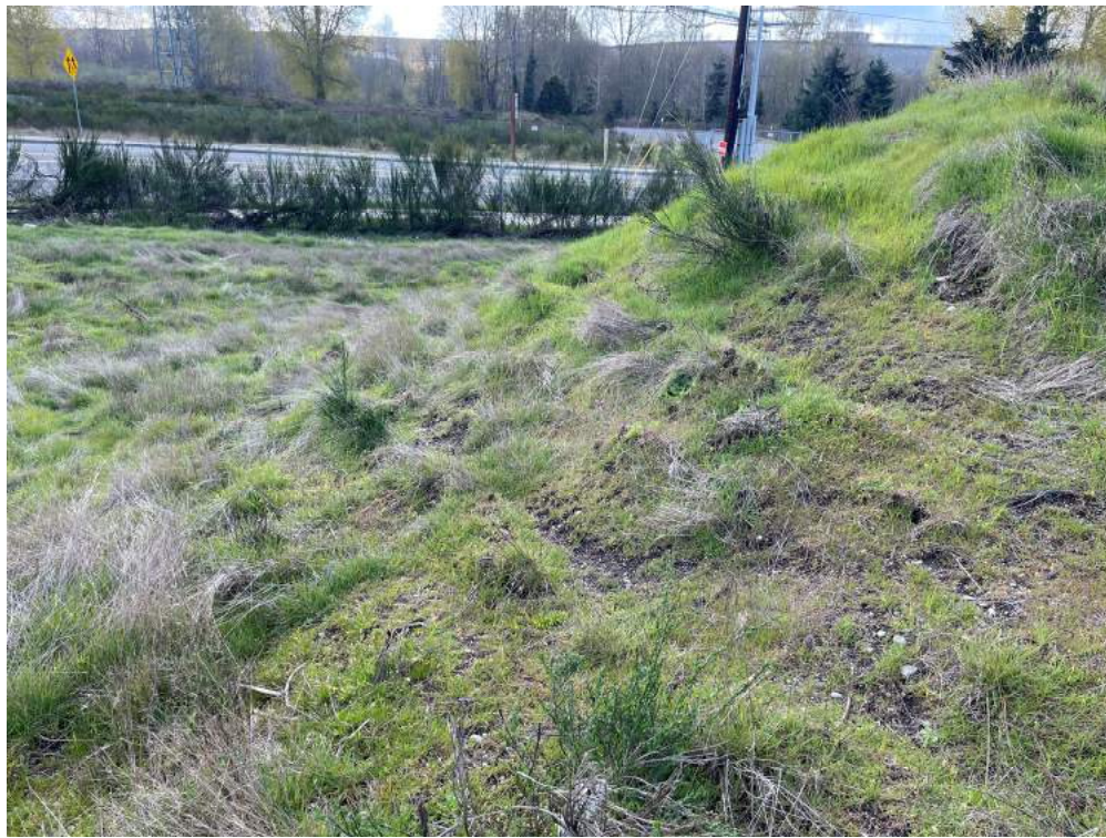
Photograph L1. Station LLA 02 showing vegetation loss and exposed soil along the slope.
