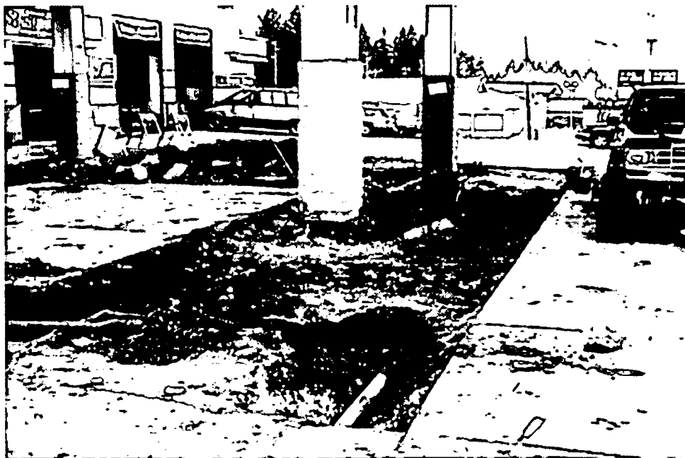
PHOTO 2: West pump island as viewed from North. Former location of diesel dispenser is in the foreground.
