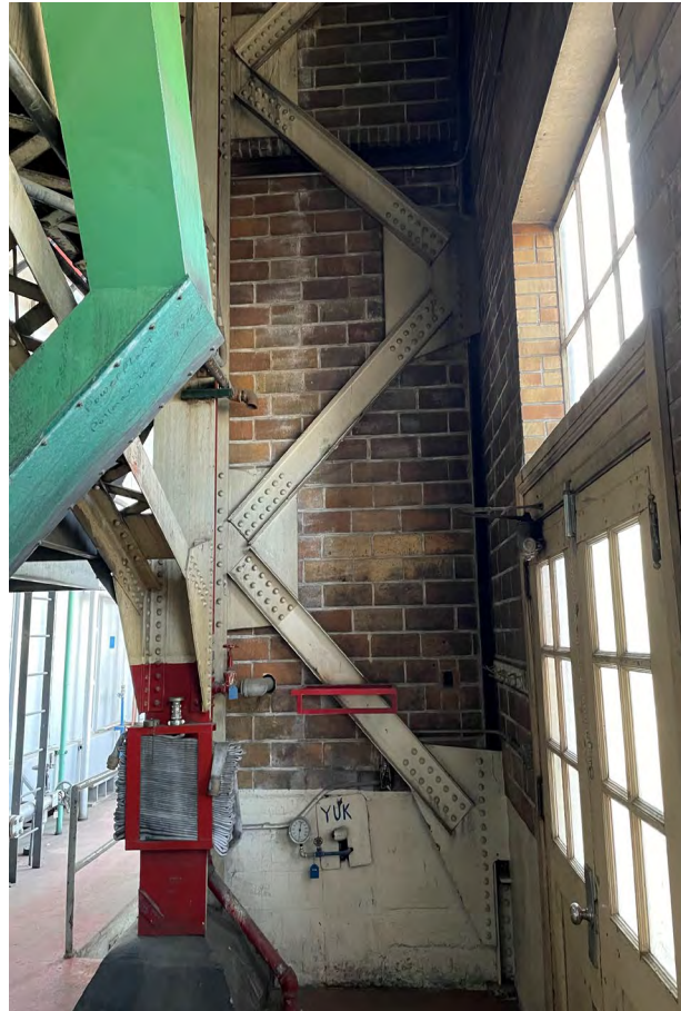
Figure 10: Interior Bracing Photograph
